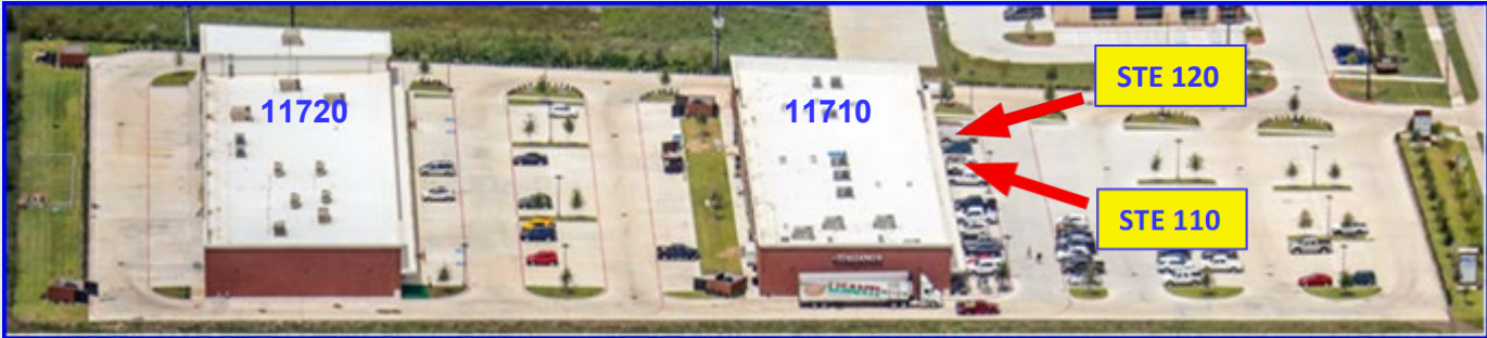
CONCRETE, WELL-LIT PARKING - 300 SPACES, 6.3 / 1,000SF RATIO
