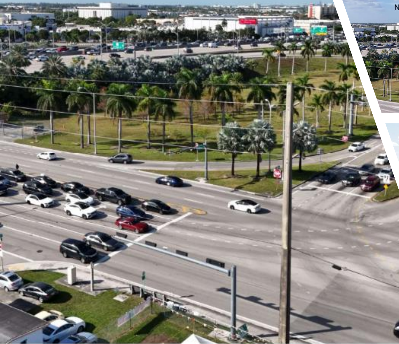
NORTH-WEST VIEW - 826 HWY
