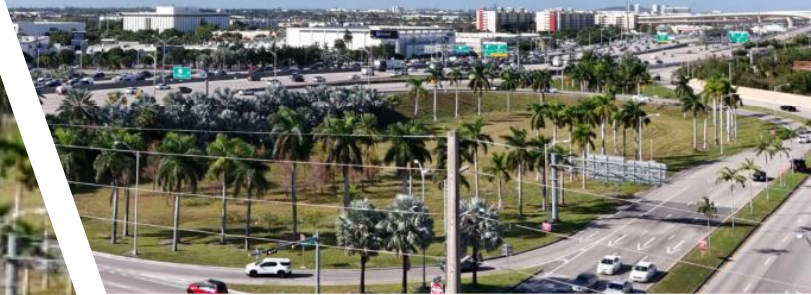
NORTH-WEST VIEW - 826 HWY
