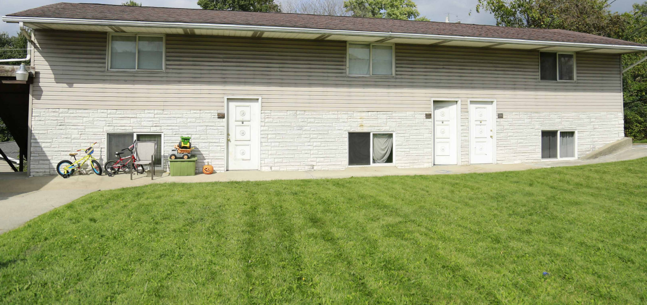
Building C - Exterior.
