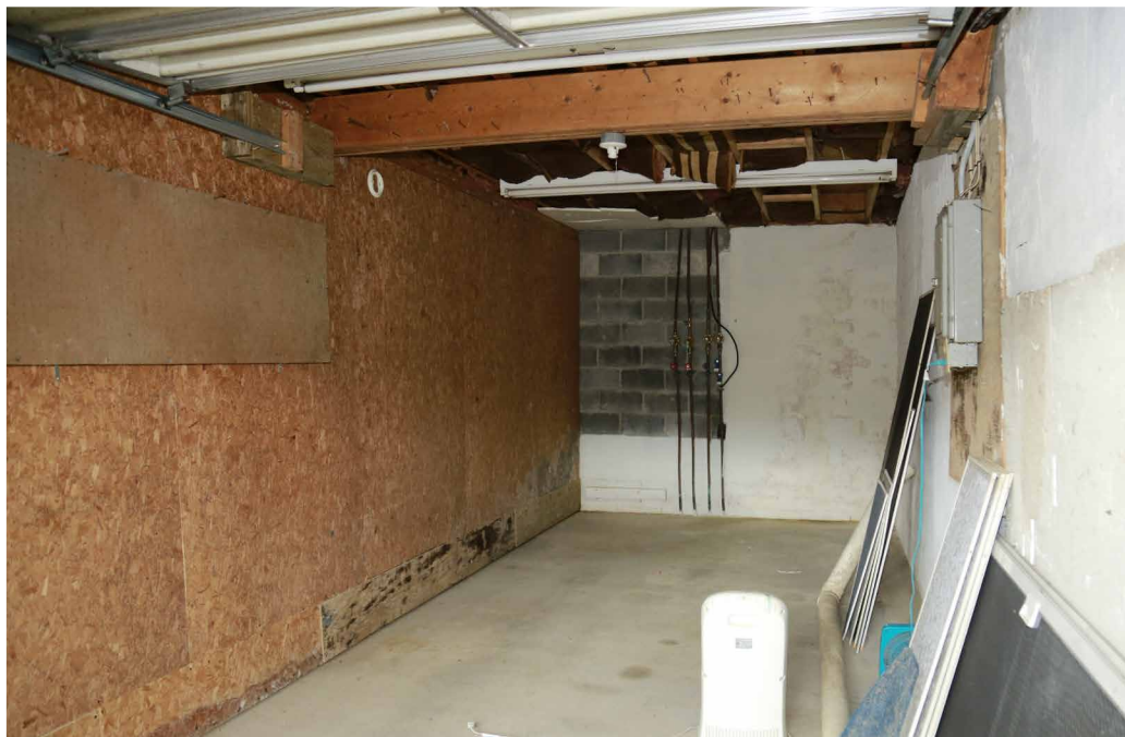
Building A Garage.
