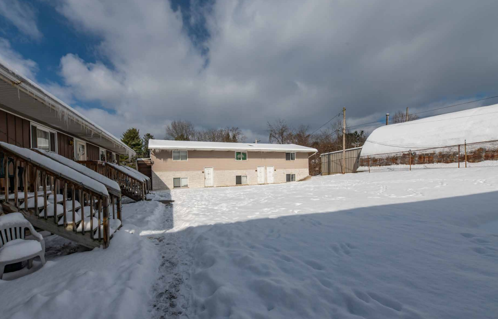
View of Building C from the Courtyard.
