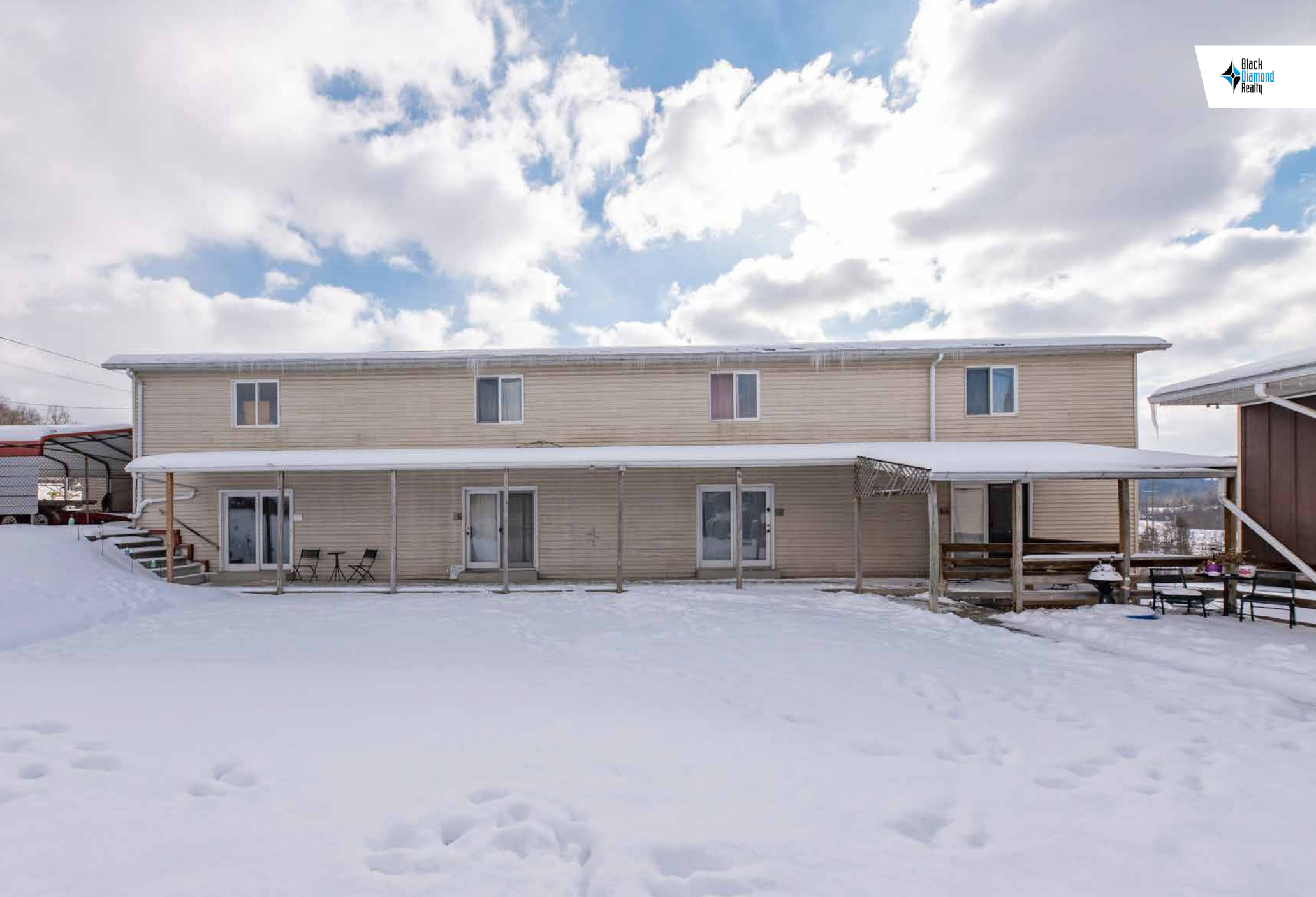
Building A - Exterior.
