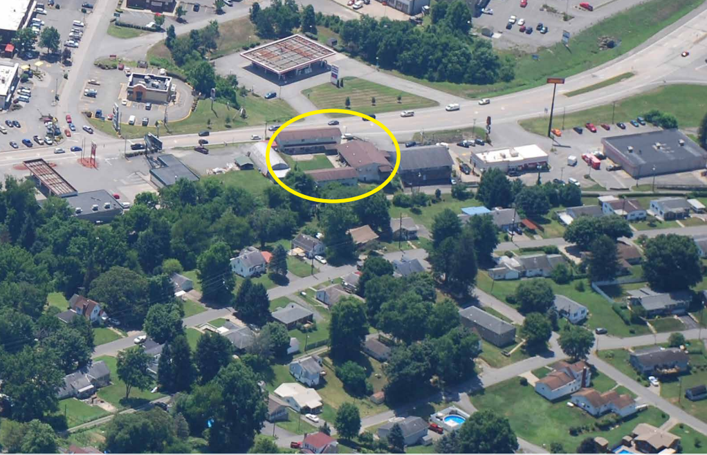
View of the Property Facing South.
