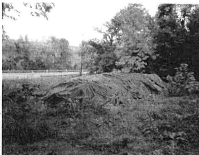
Photo 34 (10/3/2013): After the soil pile had been sampled, it was completely re-covered with 6mil plastic and secured.
