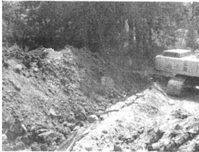
Photo 12 (8/30/2012): On-site soil treatment pile prior to being covered with 6mil plastic.
