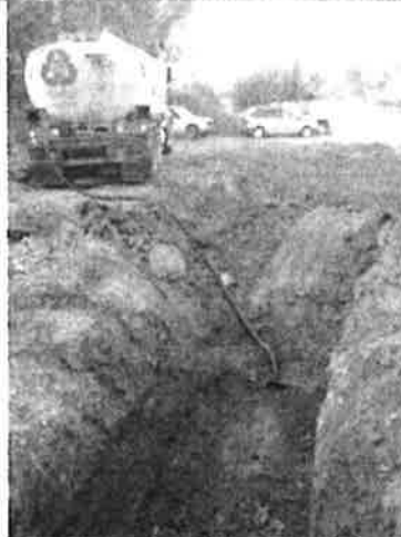
Photos 13,14, 15&16 (8/31/2012): An unregulated steel UST of approximately 550-gallon capacity was discovered north of the primary excavation area by following a steel product line from the former dispenser island. The tank contained water free of any signs of petroleum product, which was evacuated by Environmental Specialists, Inc. The tank was removed and exploratory digging was completed to a depth of 8 feet below grade in the area north of the primary excavation area. Soil screening samples were collected throughout the area. No additional tanks were encountered.
