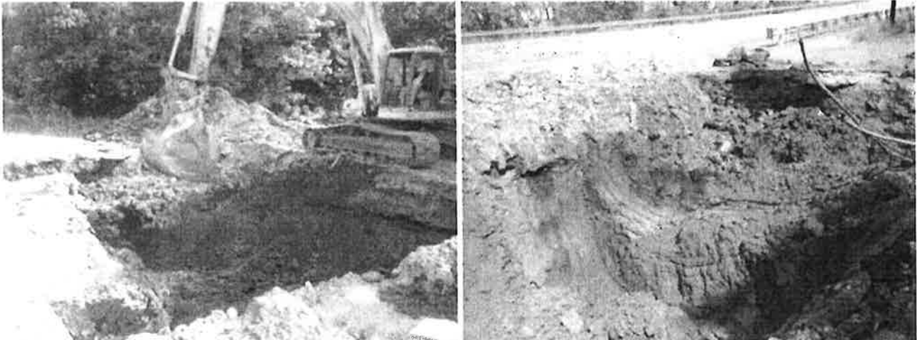
Photos 9&10 (8/30/2012): Soils 3 to 9 feet below grade across the excavation generally exhibited indications of significant petroleum impact such as staining and strong vapors; they were dug out and added to the contaminated soil pile for on-site treatment.
