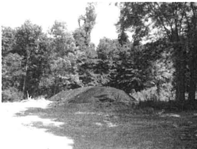
Photos 19&20 (8/31/2012): The stockpiled soil was covered with 6mil plastic to allow for air movement below the plastic and to prohibit rainwater or runoff to infiltrate the pile.
