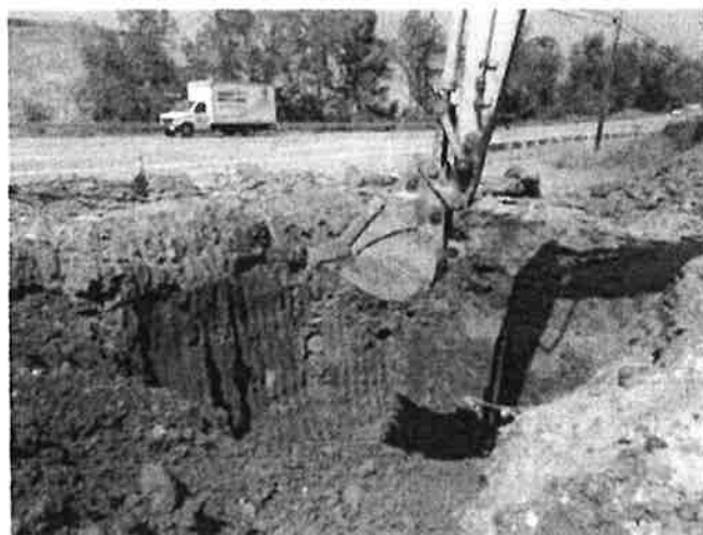
Photo 12 (8/30/2012): Soil samples were collected from the sidewalls of the excavation at 10-foot intervals with a bias toward the most obviously contaminated.
