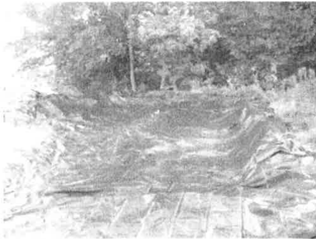
Photos 5&6 (8/30/2012): 6mil plastic was laid across the entire bottom of the stockpiling / soil treatment area and up the berms to contain any liquids from leeching through the stockpile into the subsurface.
