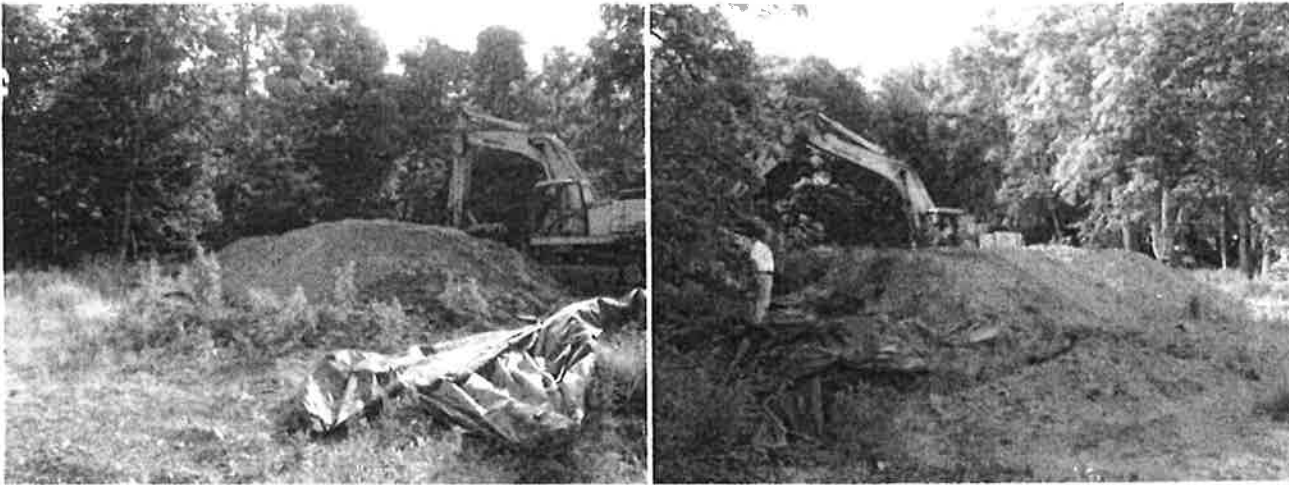
Photos 26&27 (6/25/2013): The soil pile appeared free of visual signs of contamination before it was completely turned and moved to Treatment Cell Location B.
