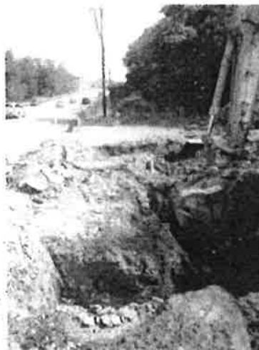
Photo 8 (8/30/2012): The western extent of the excavation was moved 4-6 feet to the east due to proximity to utilities near the edge of the highway.
