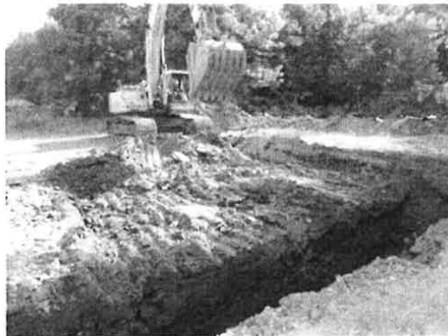
Photo 7 (8/30/2012): To commence excavation activities, the top 20-36 inches of gravel and clean material from the proposed area were removed. Some of this material was used to create a berm between the excavation and Washington Road; the remaining material was added to the "presumably clean soil pile".
