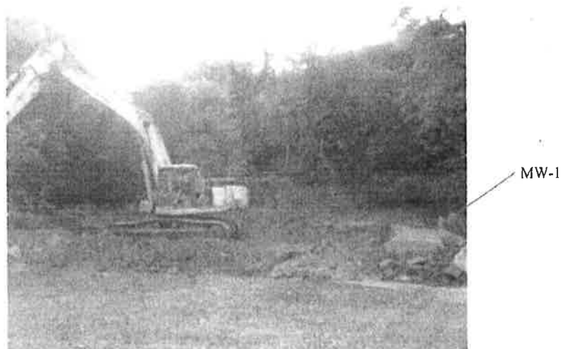
Photo 4 (8/30/2012): Preparation of the stockpiling / soil treatment area: an area measuring approximately 40 feet by 30 feet was graded level and surrounded with an earthen berm approximately 30 inches high.
