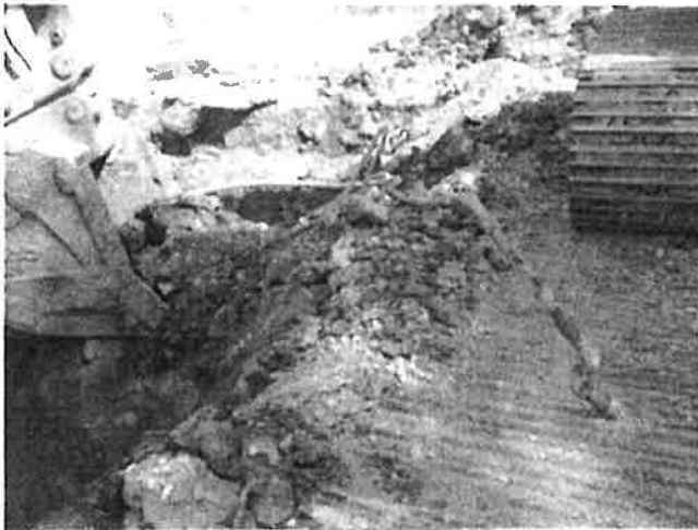
Photo 12 (8/30/2012): On-site soil treatment pile prior to being covered with 6mil plastic.
