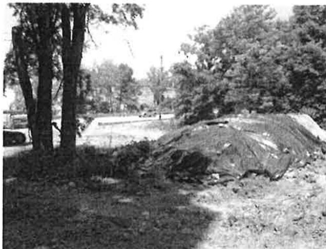
Photo 31 (6/25/2013): After the soil pile had been completely turned and moved, it was completely covered with 6mil plastic and secured.
