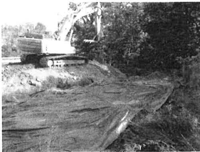
Photo 28 (6/25/2013): Showing the preparation of Treatment Cell Location B immediately east of Location A, prior to movement of the soil pile.
