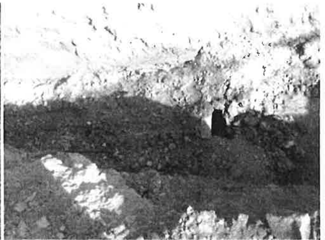
Photo 12 (8/30/2012): On-site soil treatment pile prior to being covered with 6mil plastic.
