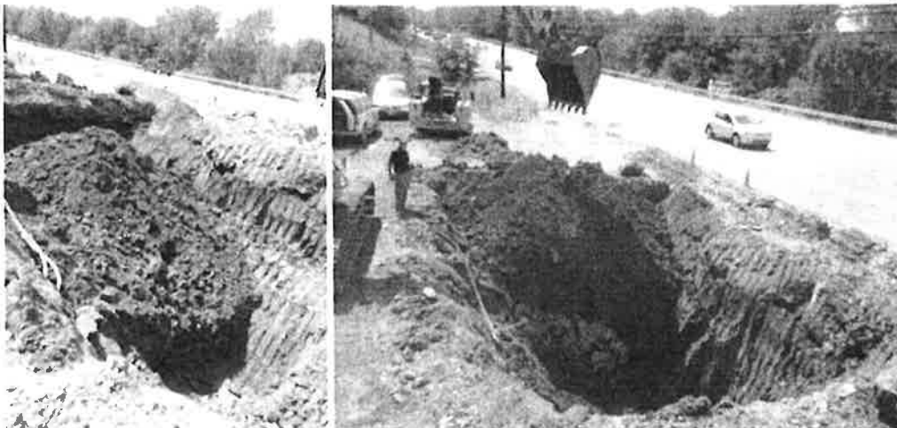
Photo 11 (8/30/2012): Soils 9 to 14 feet below grade generally did not exhibit obvious visual indications of contamination, though they did exhibit variable degrees of petroleum vapors. Therefore, soils from 10 to 14 feet below grade were dug within the excavation and completely turned over so as to release any volatile organic compounds and introduce oxygen to the subsurface to facilitate in situ remediation of soils remaining at the Site.
