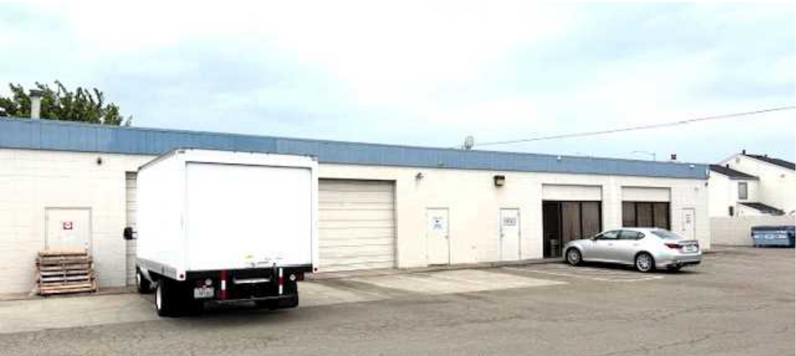
Four Warehouse Units
