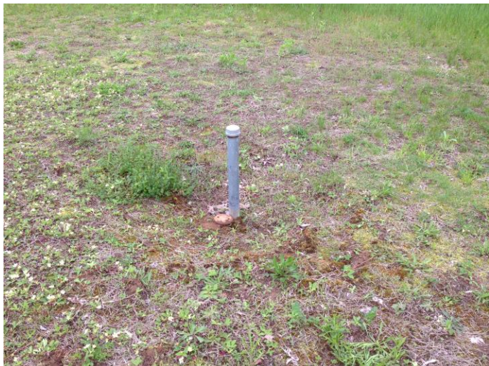
Photograph 5: View of the suspect fill pipe on the subject property.
