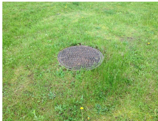
Photograph 6: View of as typical sewer manhole on the subject property.
