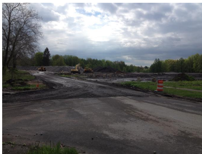
Photograph 2: View of the fill activities on the subject property.
