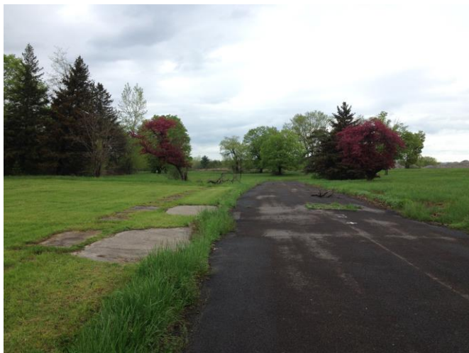
Photograph 1: View of a typical paved roadway on the subject property.
