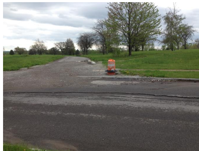
Photograph 8: View of a typical paved roadway on the subject property.
