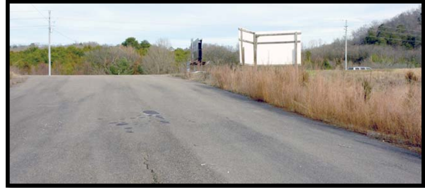
Curb Cut Entrance onto Property
