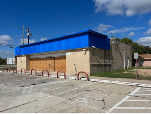
Existing 2,616 sf retail building
