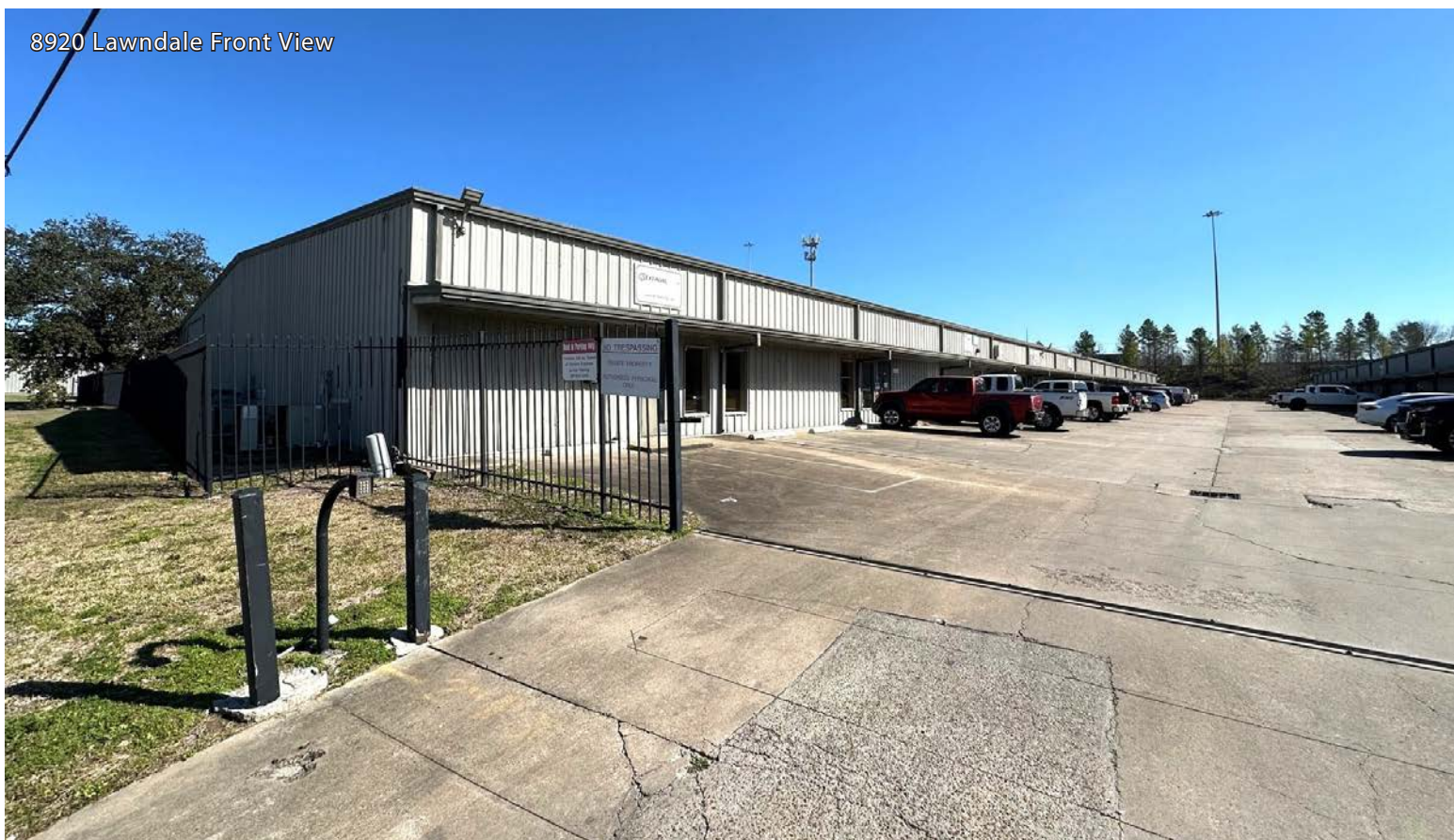
8920-A Rear Outside Storage Area
