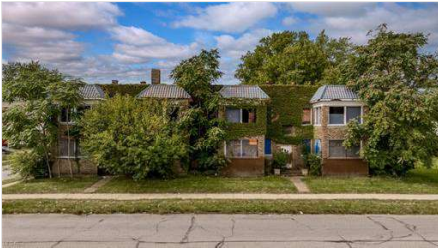
View of front facade
