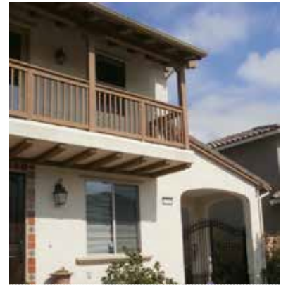
Example photo illustrating a balcony on the upper story to provide "eyes on the street."
