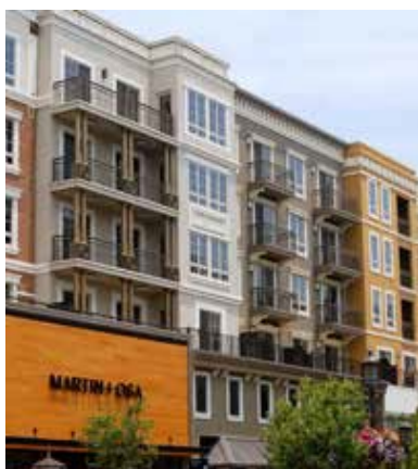
Example photo illustrating shopfront frontage type.
