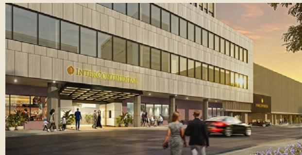
INTERCONTINENTAL This new hotel is 21-stories with 390 rooms, 20 suites, 18,000 SF of meeting space, and 4 restaurants and bars.
