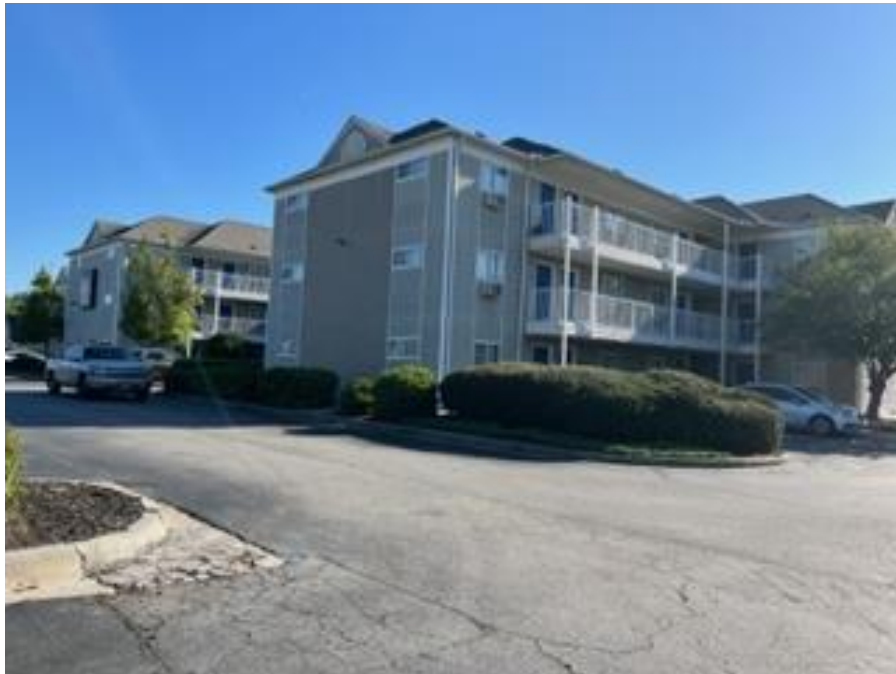
SUBJECT VIEW NORTH- INSUITES
