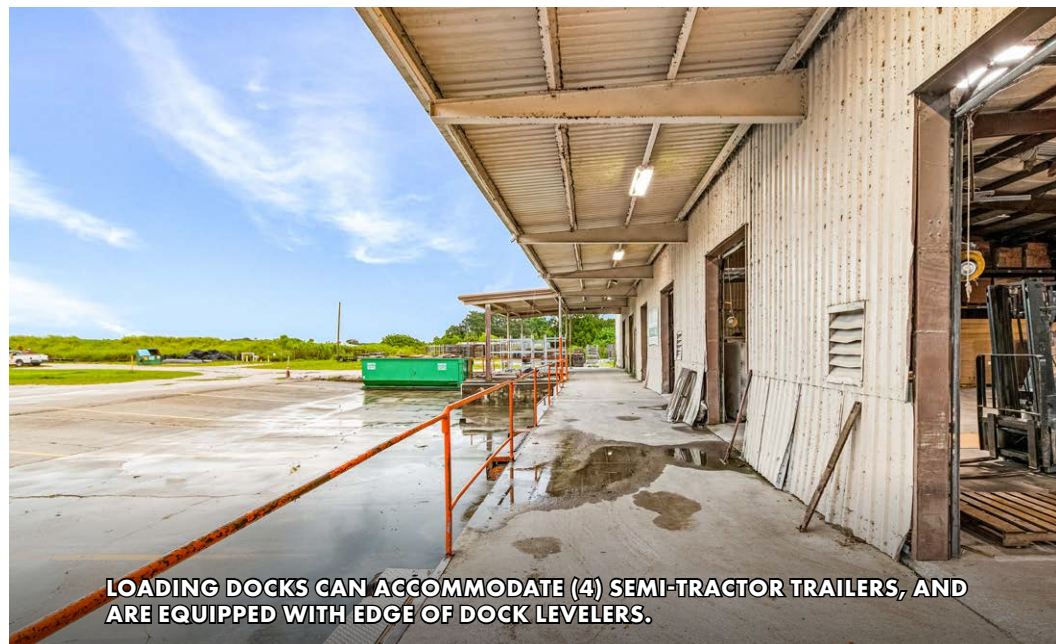
4-8' WIDE, 10' HIGH STEEL ROLL-UP DOORS PROVIDE ACCESS TO OUTSIDE COVERED LOADING DOCK
