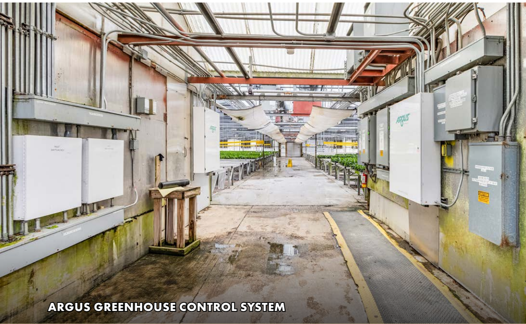
STATE OF THE ART ARGUS CONTROLS FOR AUTOMATED IRRIGATION AND FERTIGATION
