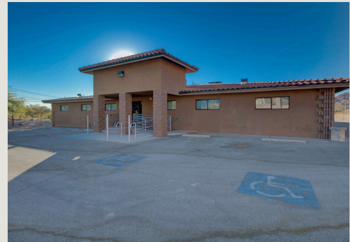
Rear entrance - upper parking lot
