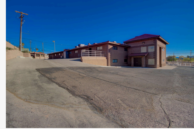
WEST SIDE VIEW
