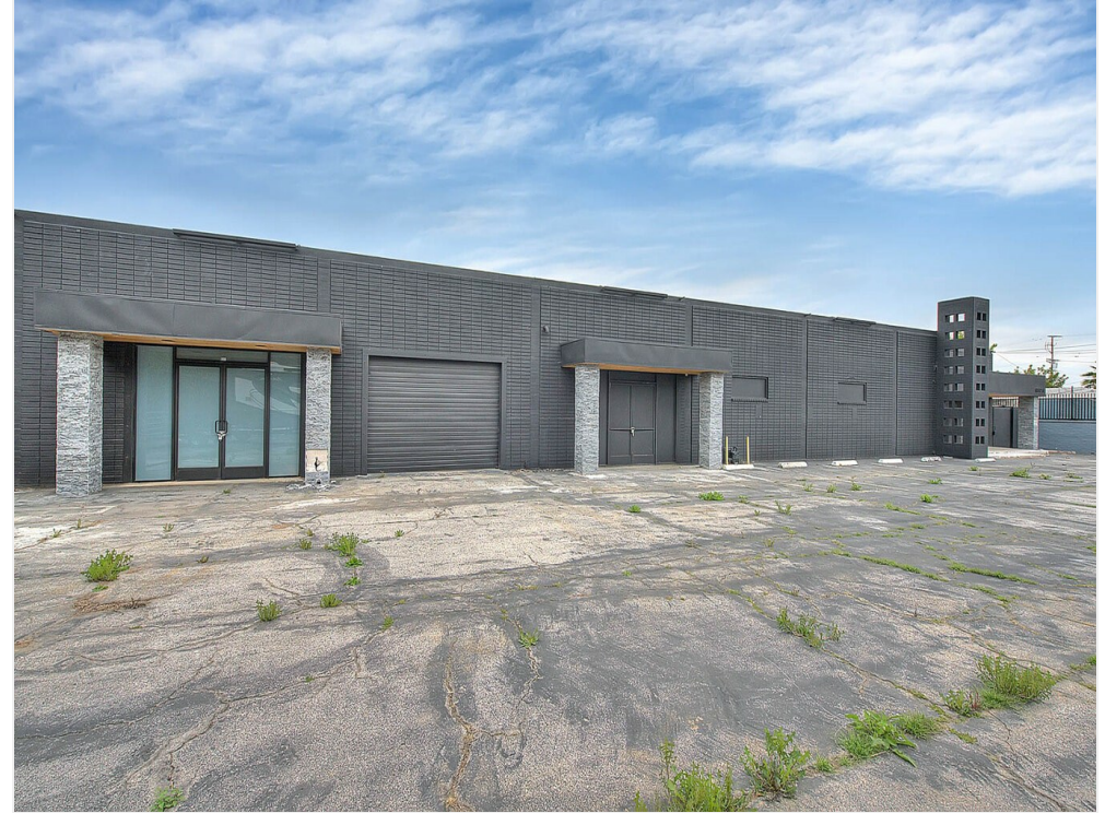
Unit 2 - Exterior (4 of 4)
