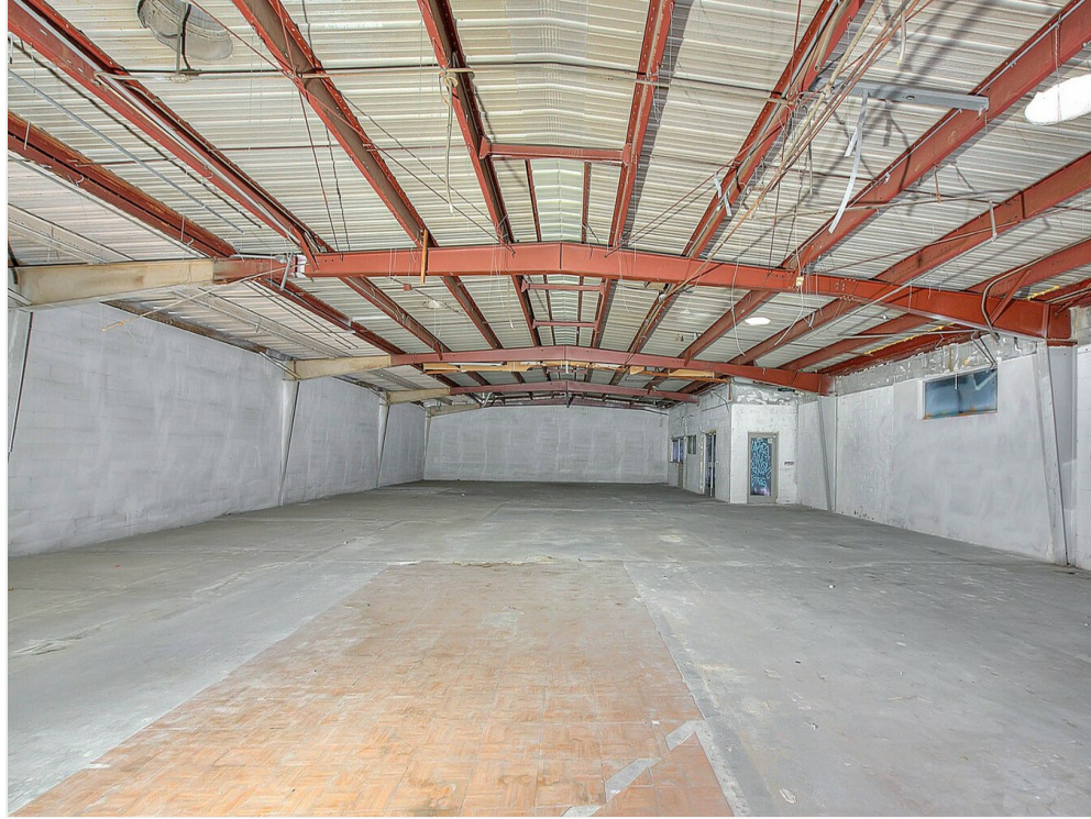
Unit 2 - Warehouse (7 of 9)
