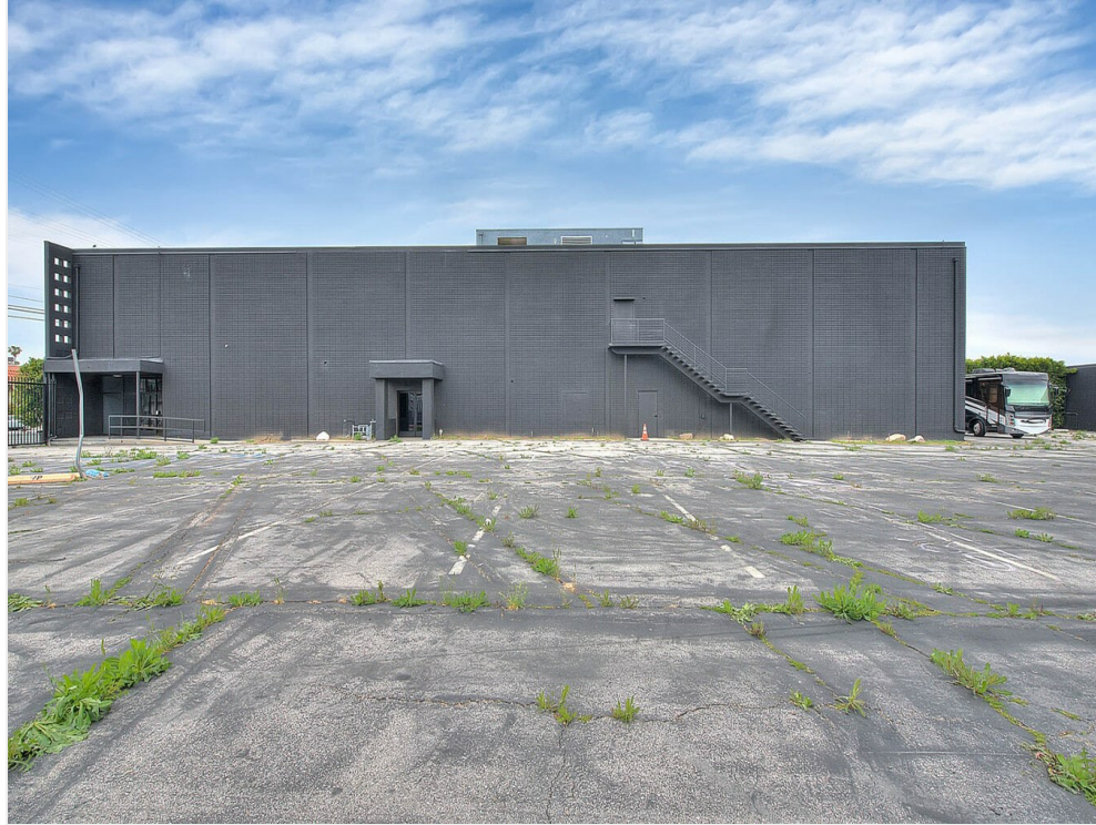
Unit 1 - Exterior View (1 of 13)
