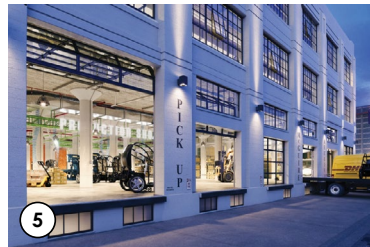
5 SECTIONAL DOOR/LOADING DOCK
