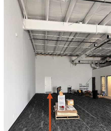
Added man door connecting Space #1 and #2
