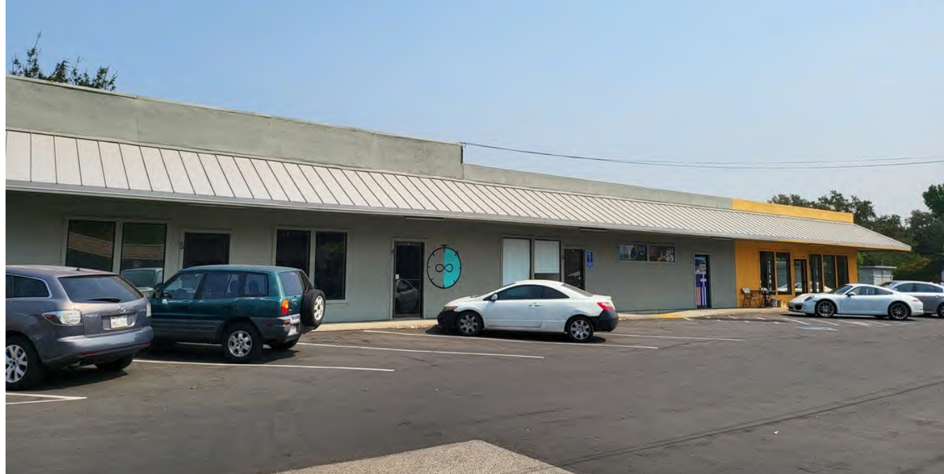
SIDE OF BUILDING
