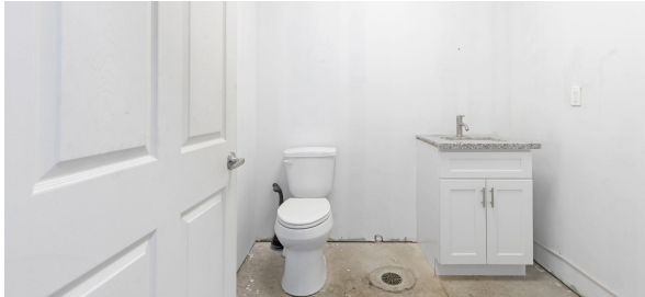
Warehouse Interior View
