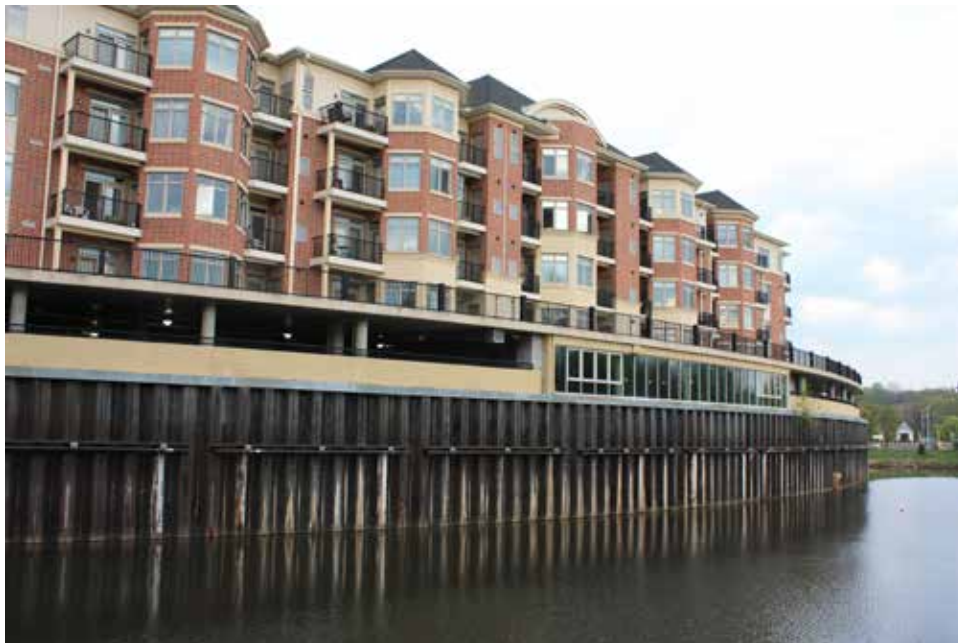
Elevated Structure, Pennypack Creek
