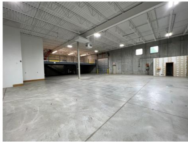
Large warehouse space with (14'Hx12'W) drive-in door and 19'6" clear height.
