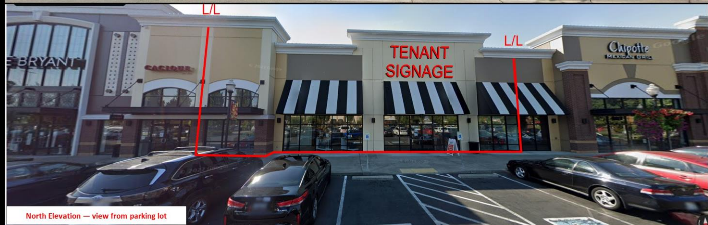
North Elevation — view from parking lot
