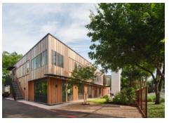
Designed by Mark Odom Studio, 4000 Medical Parkway is a 2023 renovation of a 70s office building into a creative studio with increased functionality and aesthetics. A unique triangle-shaped structure reimagined with a high performance thermo-spruce facade; new skylights & windows; addition of elevator, second level glass walkway and conference room. This adaptive-reuse project also incorporates greenscapes with a welcoming "front yard".
