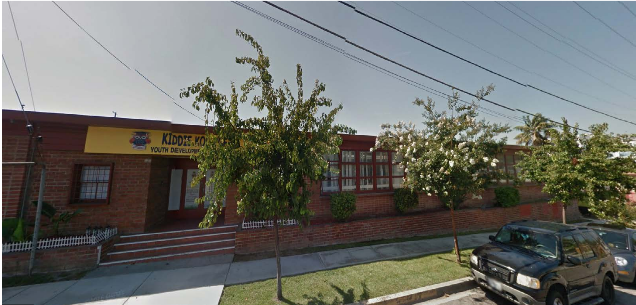
FAITH LUTHERAN PRE-SCHOOL BUILDING 3329 W. 85 TH STREET, INGLEWOOD CA 90305
