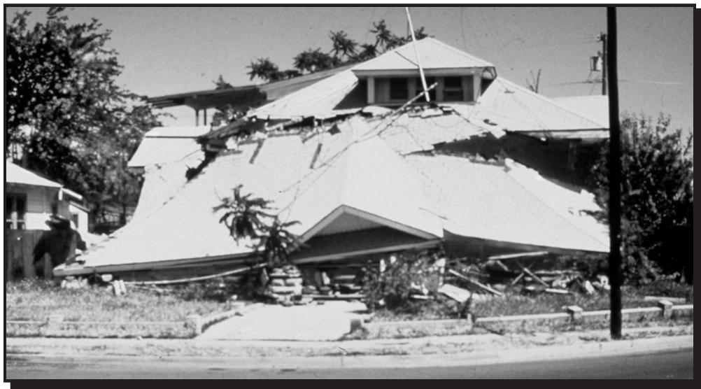
Additional damage from aftershocks
