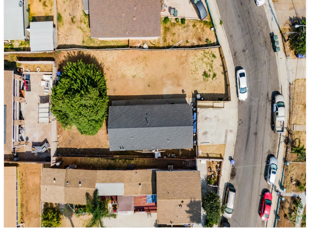
Building Photo - Aerial Neighborhood
