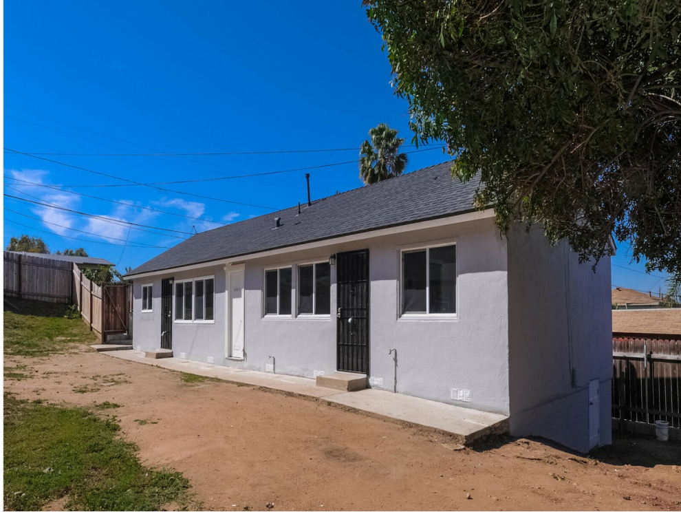
Exterior - Duplex & Laundry Room (middle door)
