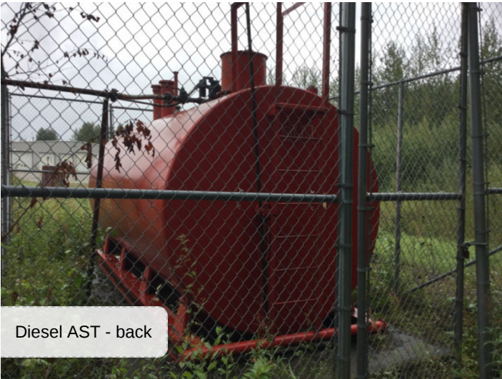
Diesel AST and fencing
