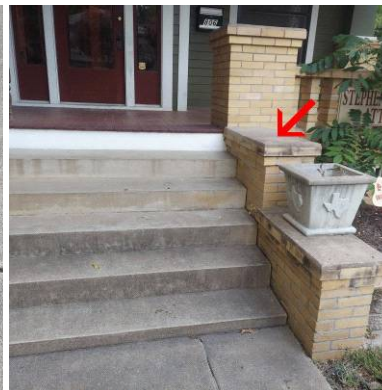
No handrail on front steps
