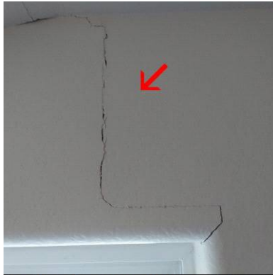
Settling fracture over up SW office window
