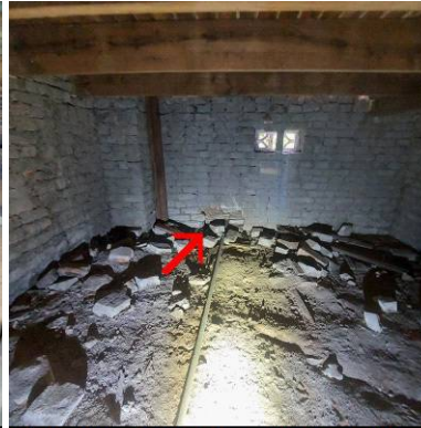
Damage to block wall in south crawl space
