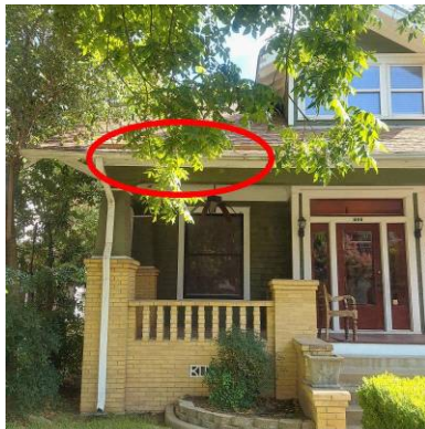
Sagging at front gutter toward west end
