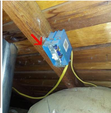
Missing faceplate at attic receptacle
