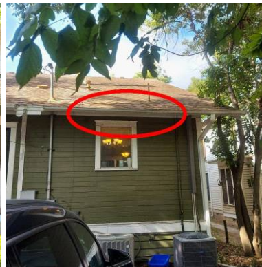
Sagging of gutter at rear west end
