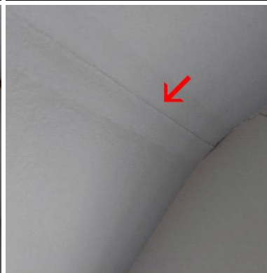
Tapeline fracture in SW office coffer
