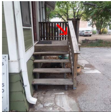
No proper handrail at patio steps
