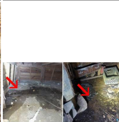
Water entering and ponding in crawl space
