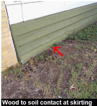
Wood to soil contact at skirting
