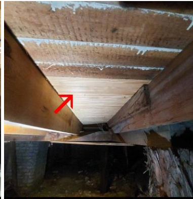
Replaced area of sub floor
