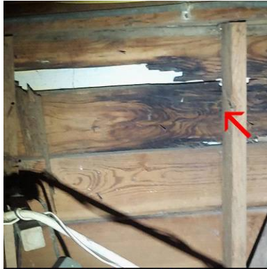
Moisture deterioration on east skirting
