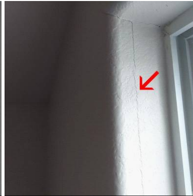
Corner bead fractures at SW office window
