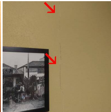
Fracture in NE office wall
