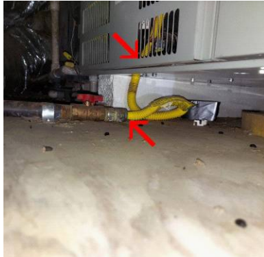
Flex line in cabinet / no sediment trap
