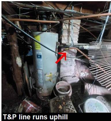
Gas valve off / no sediment trap
