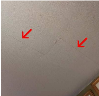
Fracture in west office ceiling
