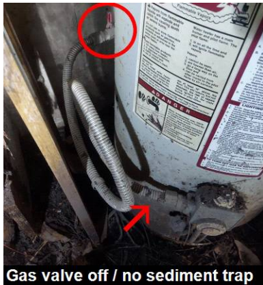
Gas valve off / no sediment trap
