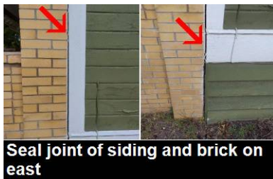
Moisture deterioration at active leak
