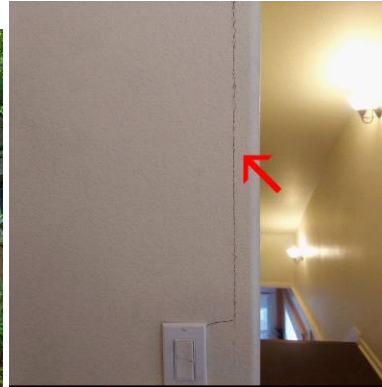
Settling fracture at upstairs corner bead
