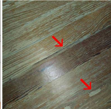
Damaged areas of hardwood flooring
