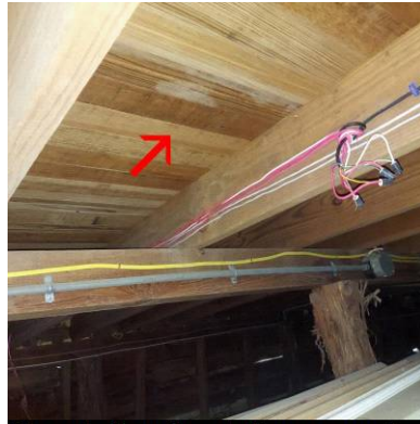
No sub floor insulation present
