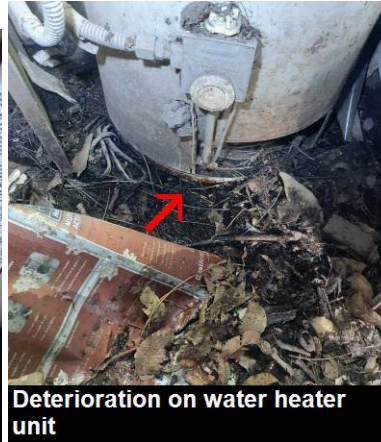
Gas valve off / no sediment trap
