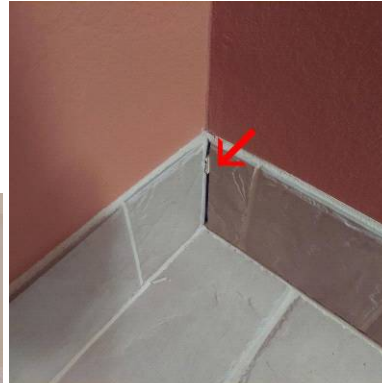
Gap in tile grout at upper bathroom
