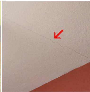
Tapeline fracture at front foyer ceiling
