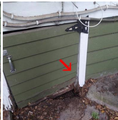
Lower hinge missing at access door
