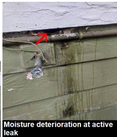
Areas of deteriorating/peeling paint
