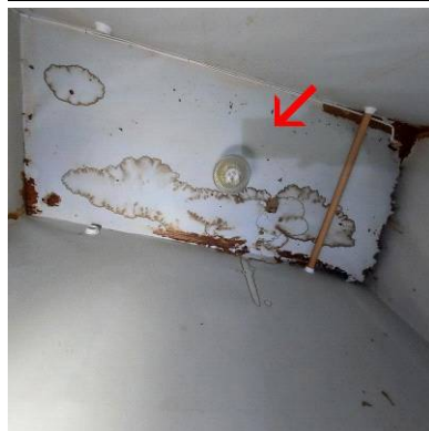
Moisture and rodent damage in closet ceiling
