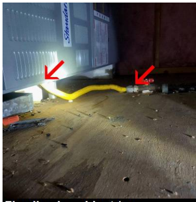
Flex line in cabinet / no sediment trap
