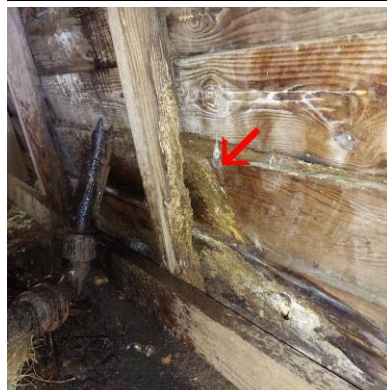
Moisture deterioration - crawl space skirt
