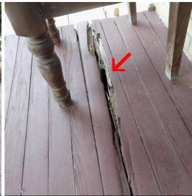
Moisture deterioration on front porch
