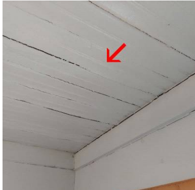
Possible moisture deterioration in ceiling
