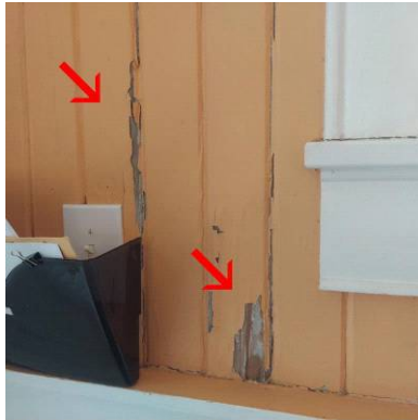
Moisture deterioration at lower NE walls
