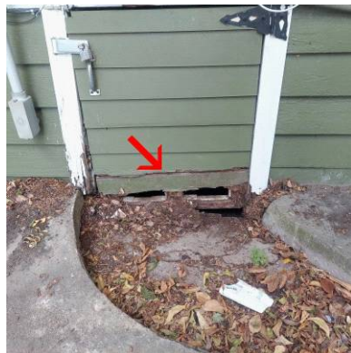
Moisture deterioration on access door
