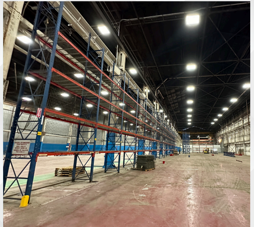
RESTORATION WORK ONGOING
