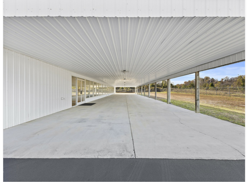
Covered Area in Front of Building
