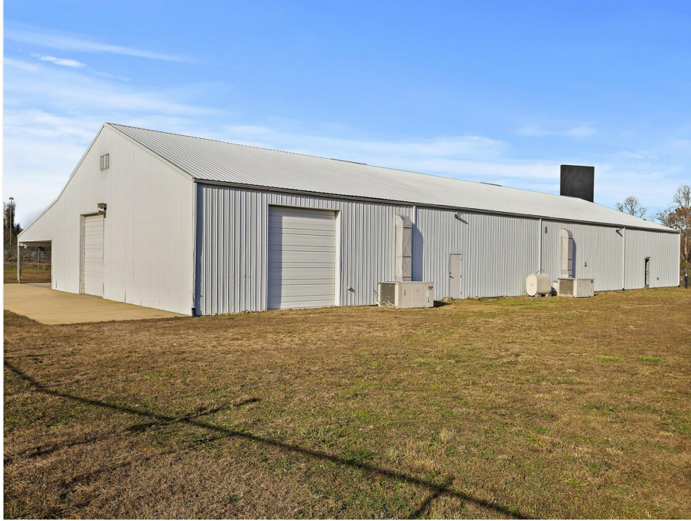
Right Side & Rear of Building
