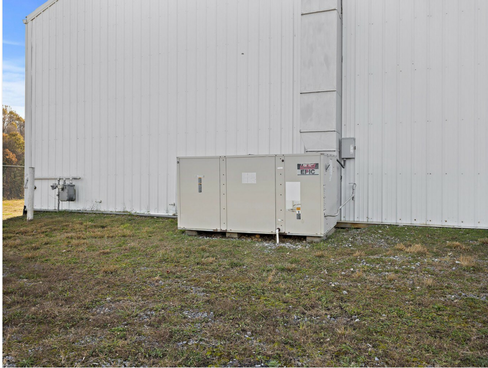
Left Side of Building
