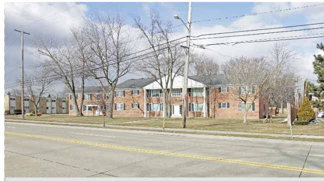
JEFFERSON AVE APARTMENTS
