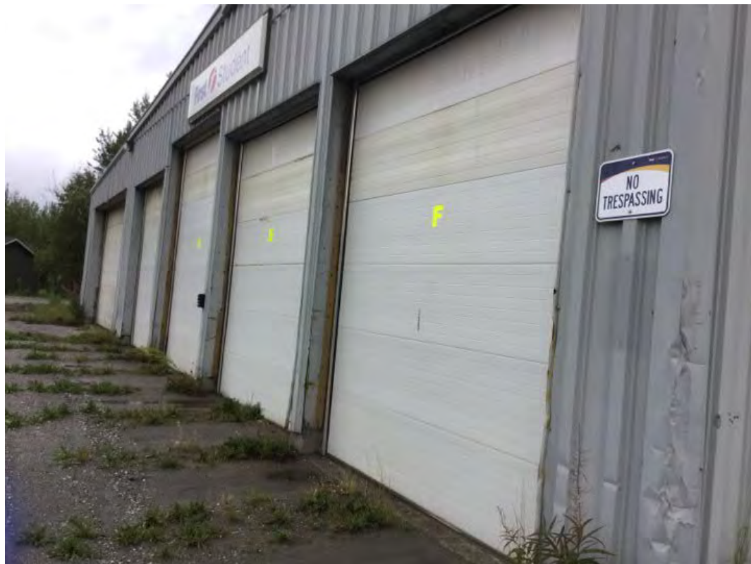
Photograph 2: Building entrance bays, west side
