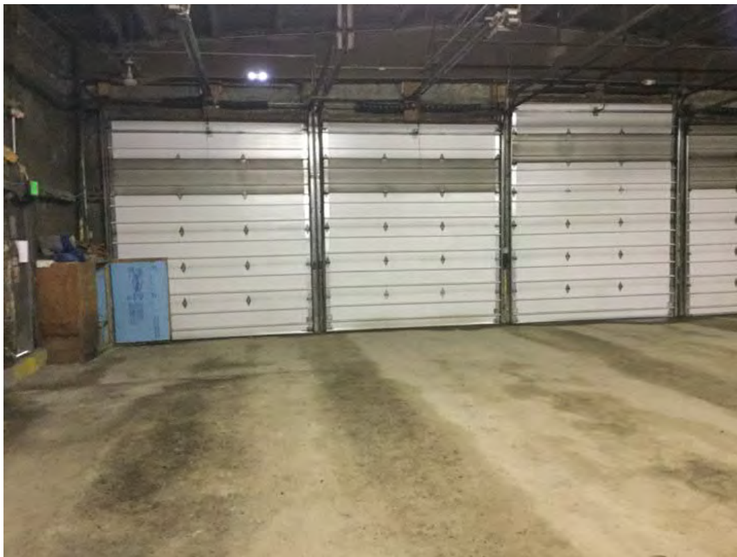
Photograph 11: West side entrance to building; municipal water meter in southwest corner
