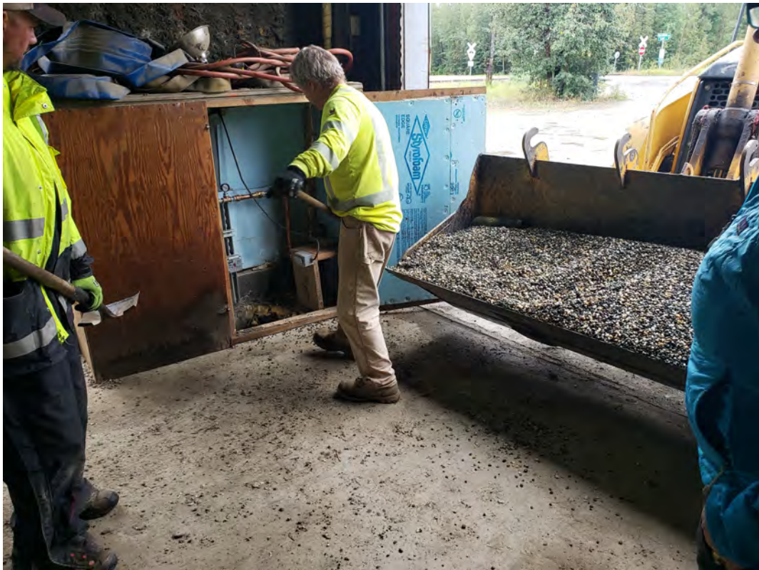
Photograph 18: Closure of former groundwater production well and new potable water meter and recirculation pump
