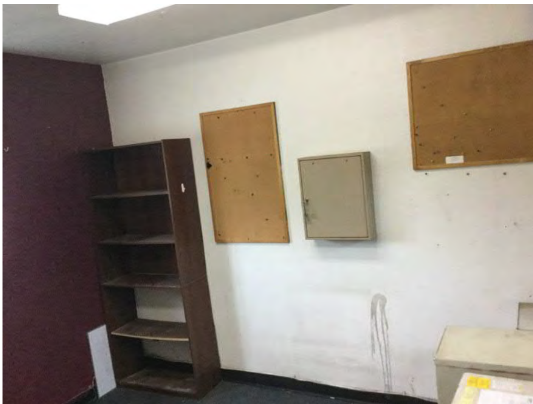
Photograph 7: Office area near main lobby at entrance
