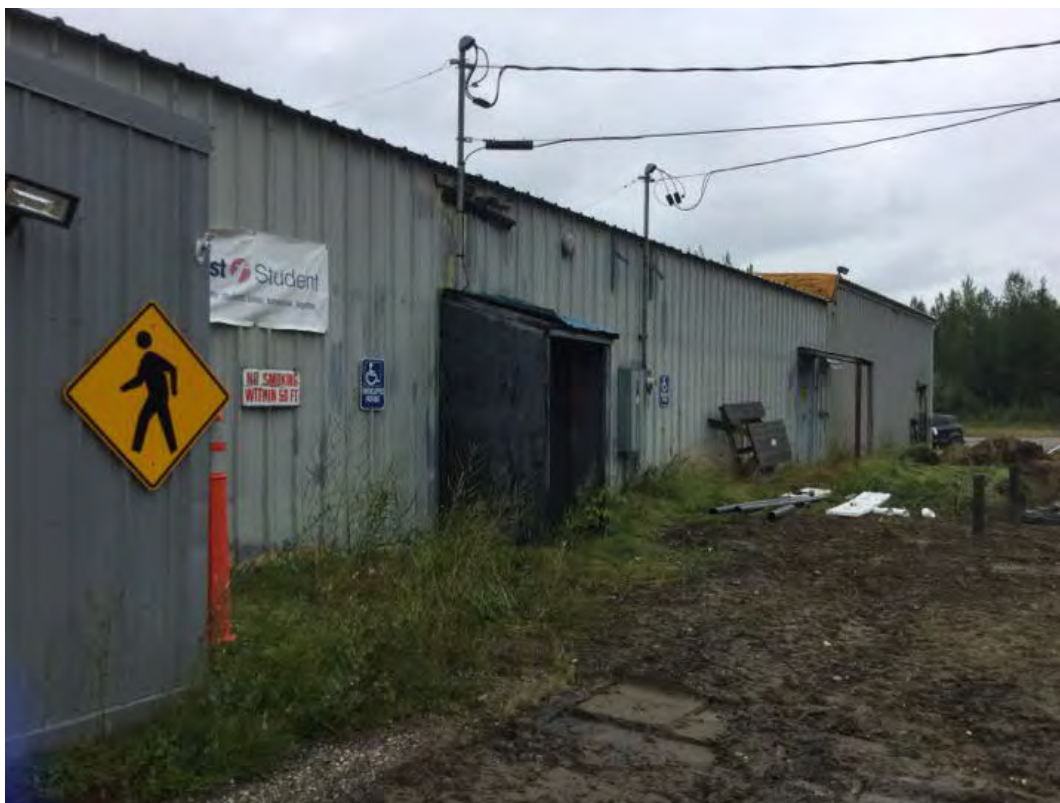
Photograph 4: Building south side (office entrance)
