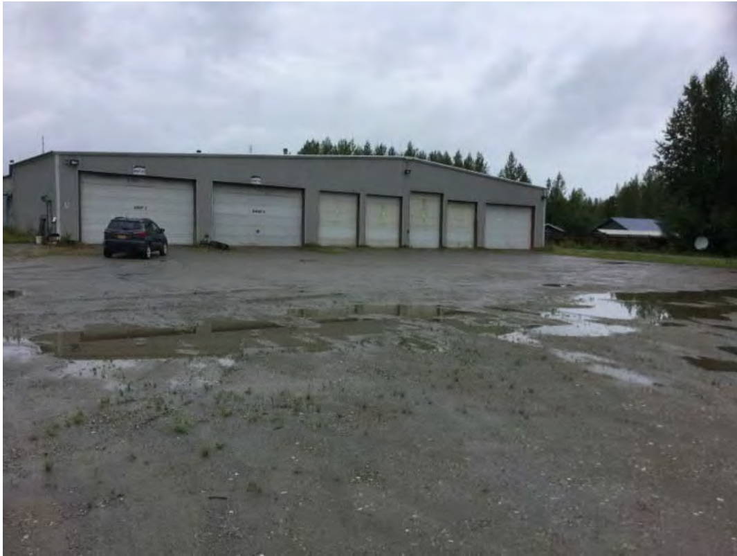
Photograph 1: Building entrance, east side
