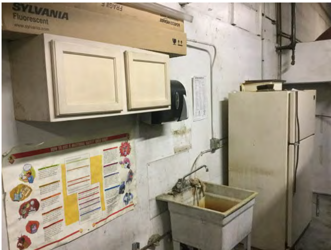
Photograph 6: Wash sink adjacent to office area and near fire water tanks
