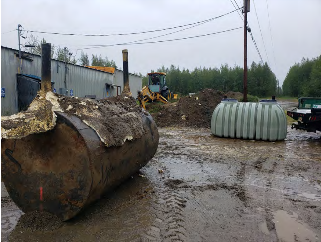
Photograph 17: Septic tank replacement project underway
