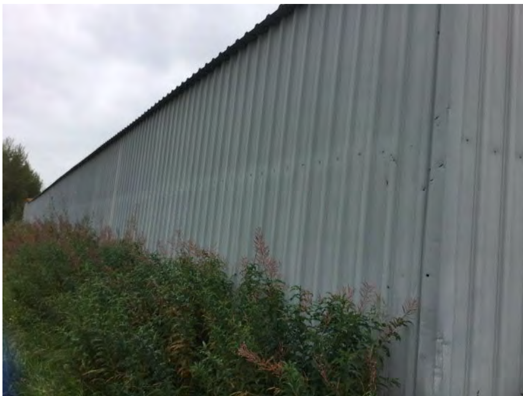
Photograph 3: Building north side
