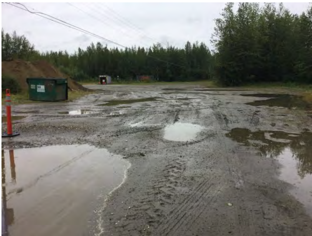
Photograph 16: Access road and parking lot, building south side
