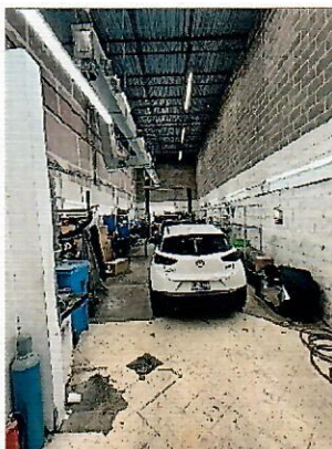
Interior view of 5707 A
