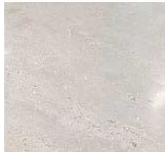
POLISHED CONCRETE FLOORING
