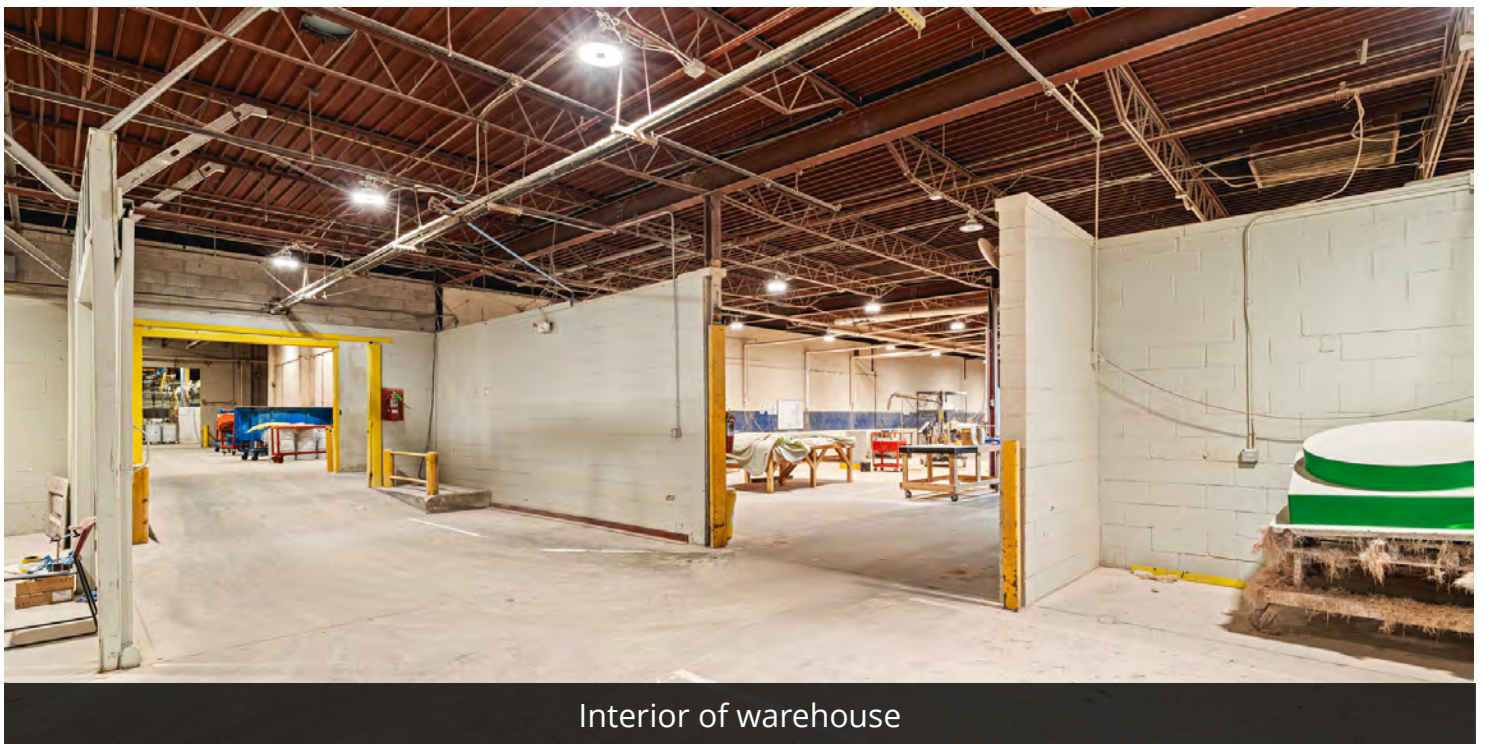
Interior of warehouse
