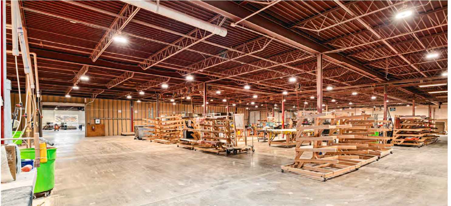
Interior of Warehouse
