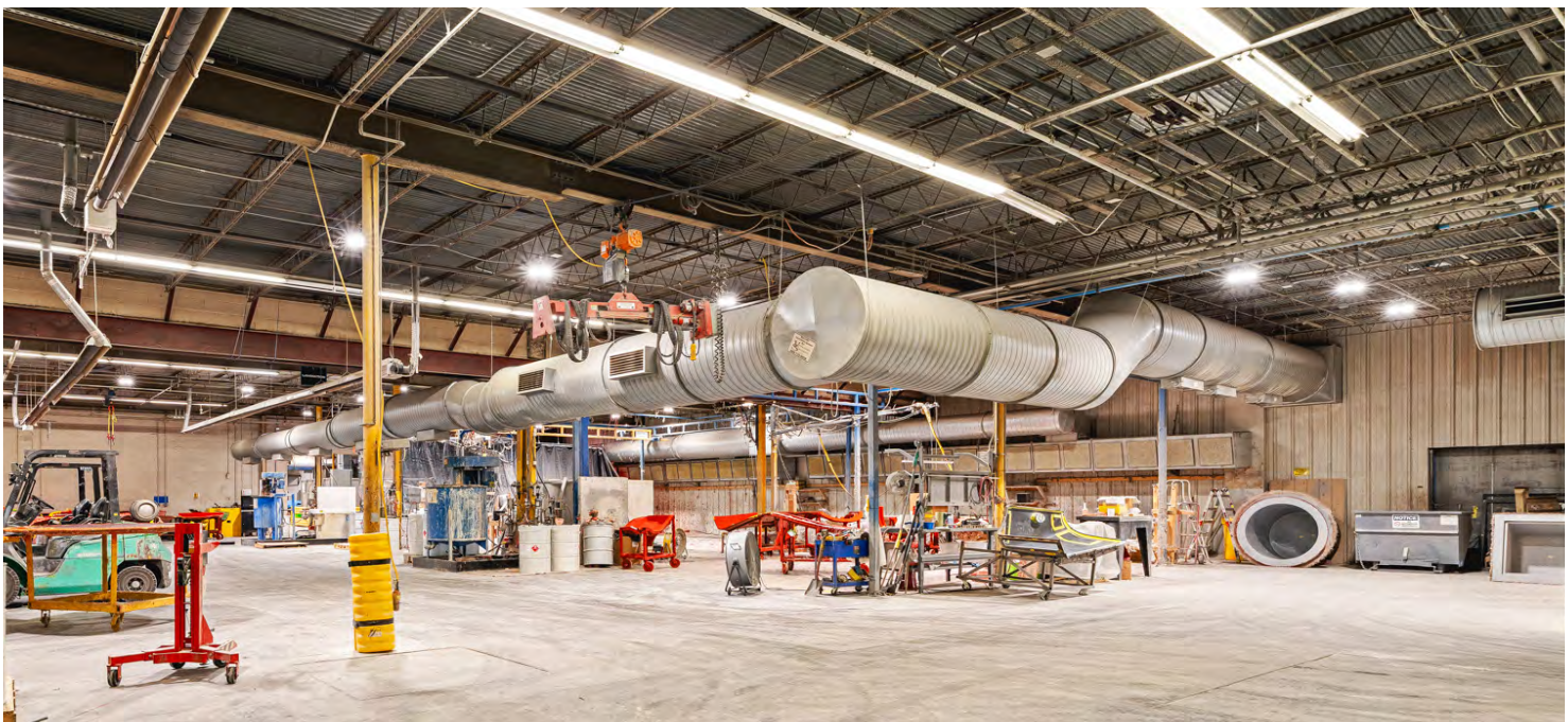
Interior of Warehouse
