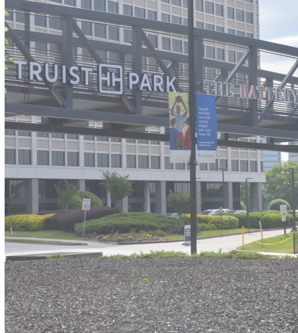
PEDESTRIAN BRIDGE FROM C75 TO THE BATTERY
