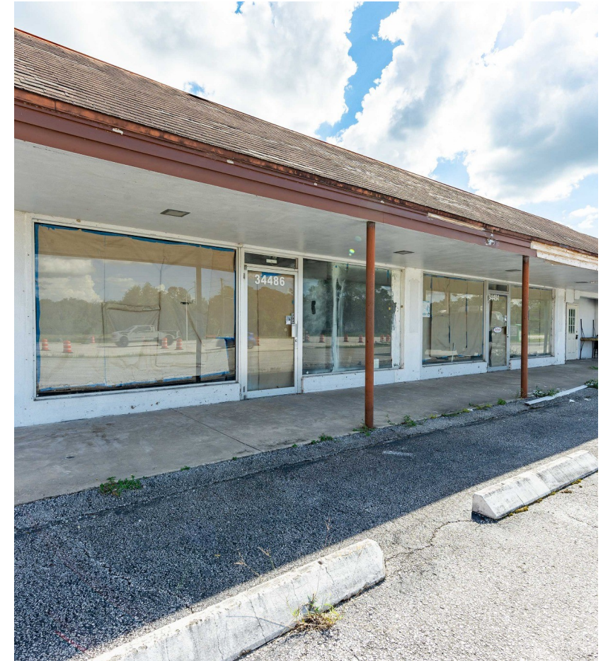
Close view of 34480 frontage
