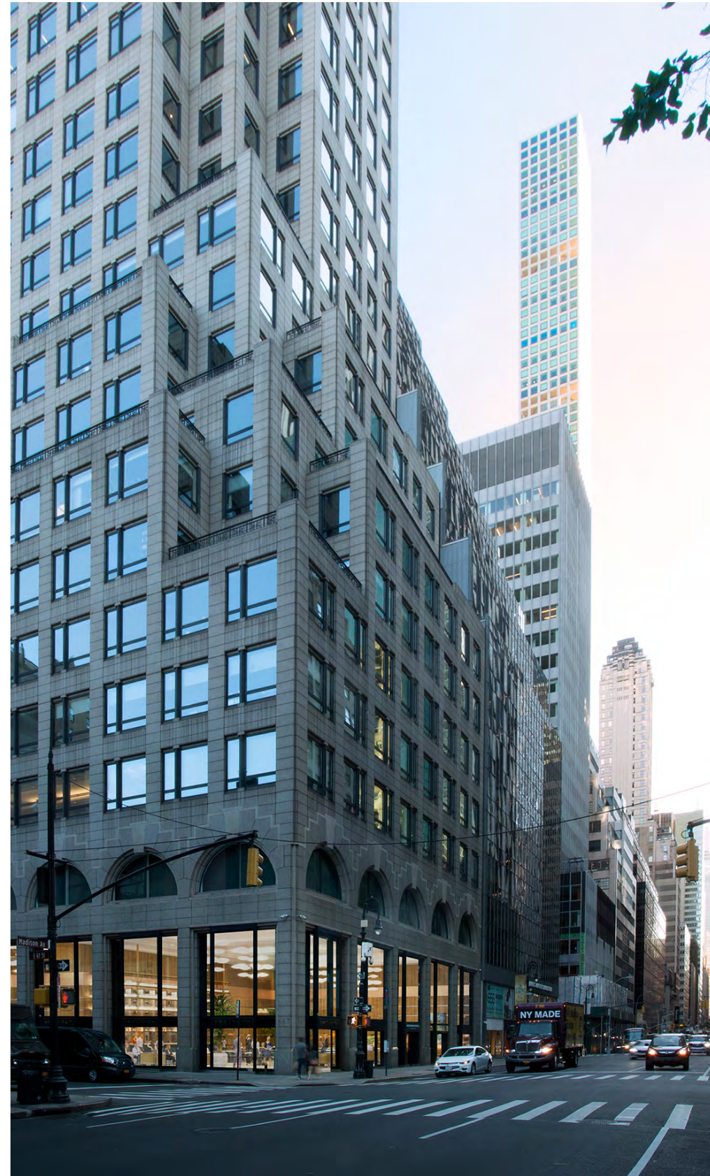
Building Northwest Corner
