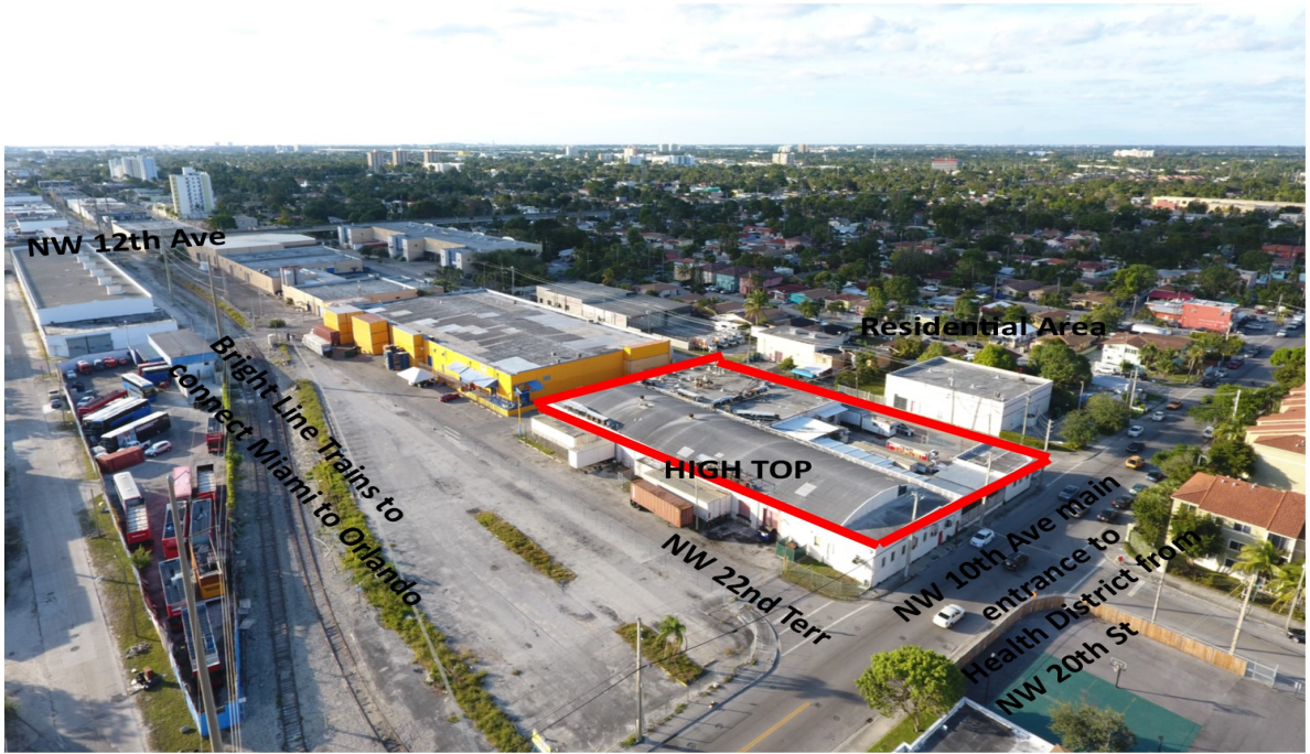
View from 12 th Ave And NW 23 rd St Looking South. Notice Proximity to Metro Rail Station
