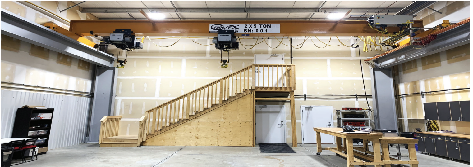
Warehouse with 10 ton crane
