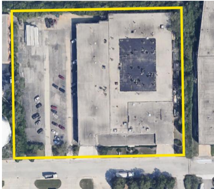
Designated inbound and outbound dock areas Building could be subdivided
