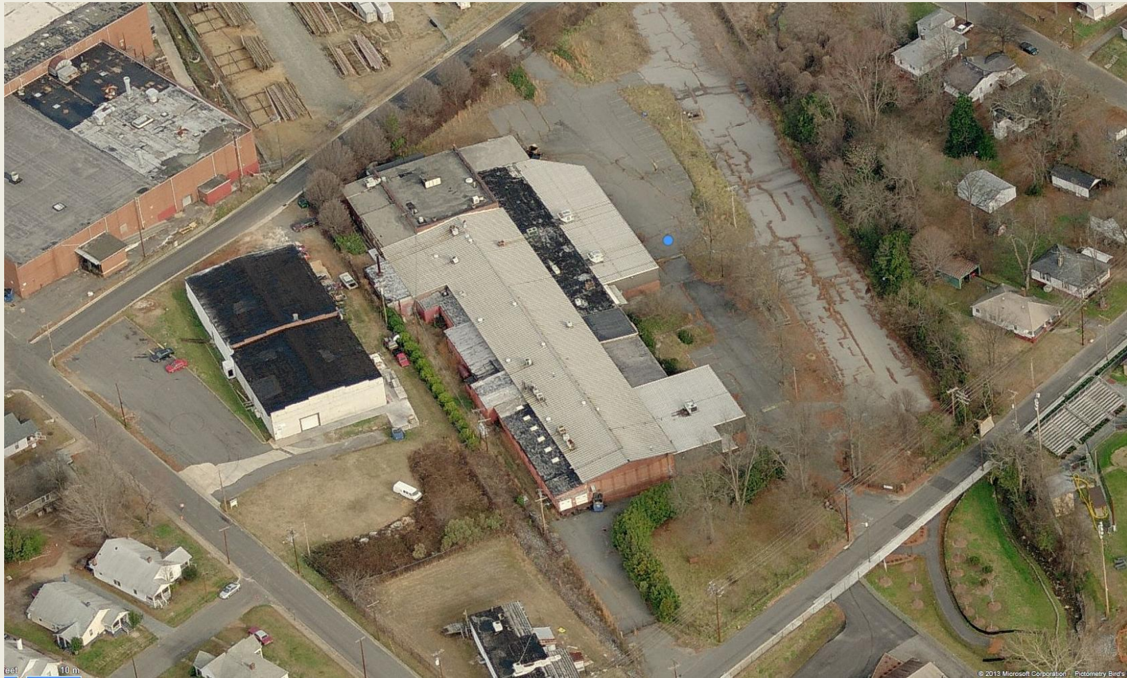
184 Academy Avenue Warehouse
