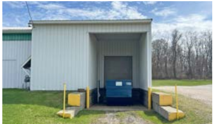
20'W x 12'H Drive-In Overhead Door & Recessed, Covered Truck Dock With 8'W x 9'H Overhead Door To Shipping / Receiving (Bay 1)
