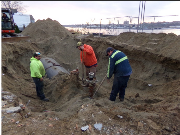
Photograph 13: Exposing 3K Diesel UST
