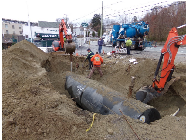
Photograph 9: Removing Soil Surrounding Gasoline UST
