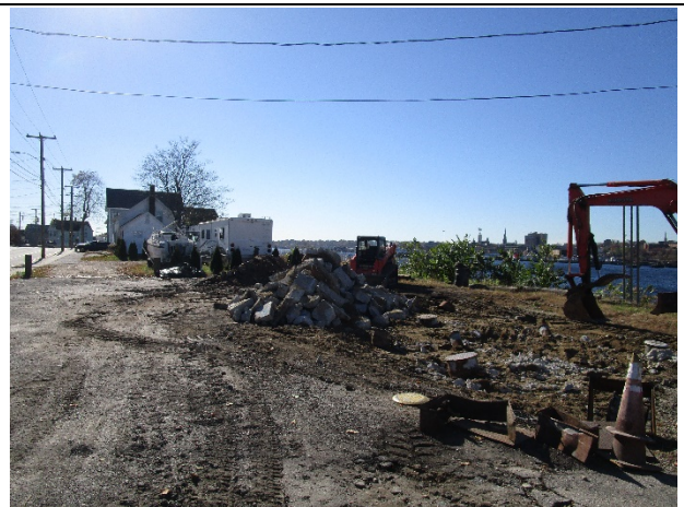
Photograph 6: Exposed UST Area
