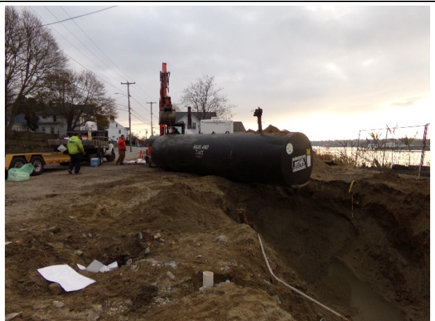
Photograph 12: Gasoline UST upon Removal
