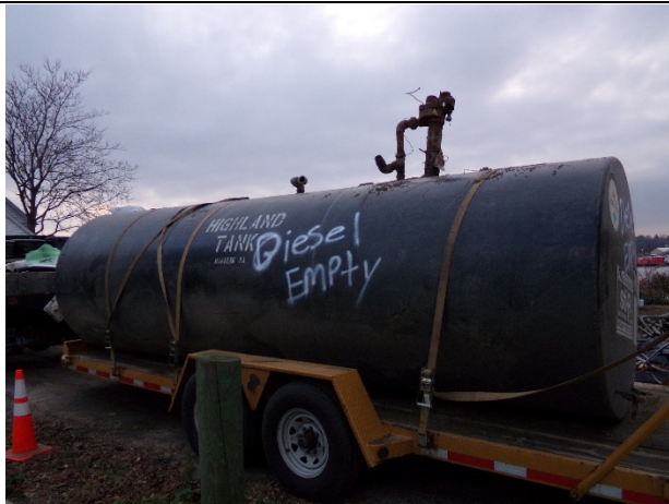
Photograph 21: Diesel Tank being Transported Offsite for Disposal
