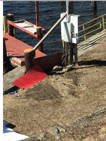
Photograph 28: Dispenser Line Area on Lower Portion of Site after Backfilling
