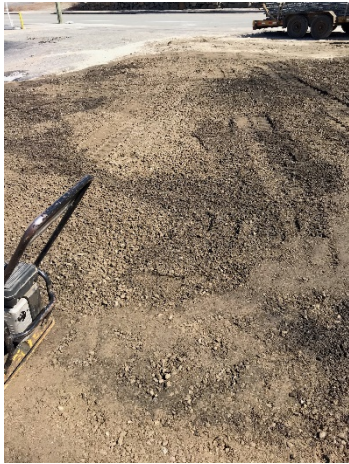
Photograph 25: UST Area after Backfilling
