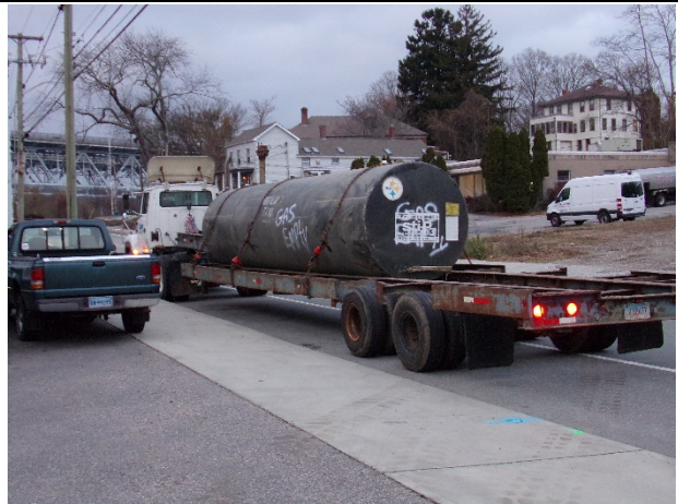
Photograph 20: Gasoline Tank being Transported Offsite for Disposal
