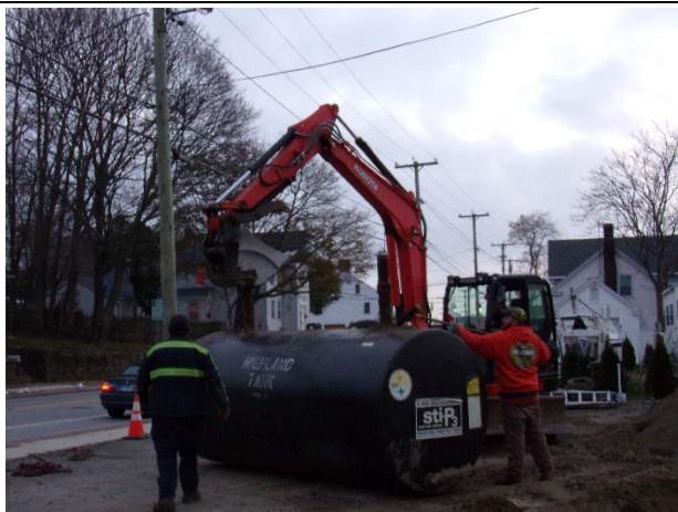
Photograph 17: 2K Diesel Tank upon Removal
