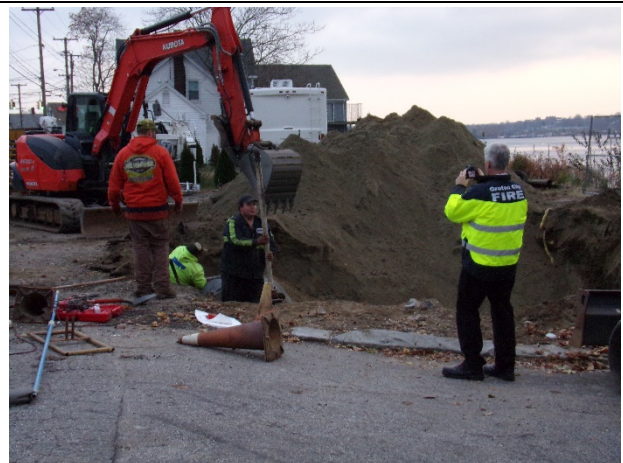
Photograph 18: Fire Marshal Observing Tank Removal Activities
