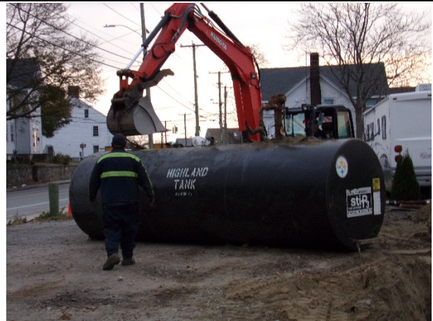
Photograph 14: 3K Diesel UST upon Removal
