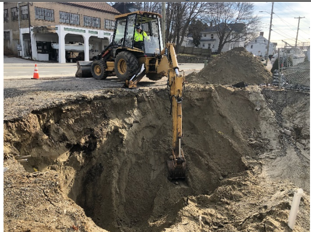
Photograph 22: Excavating Contaminated Soil
