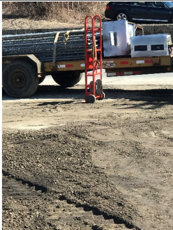
Photograph 27: Dispensers Loaded on Trailer for Offsite Disposal
