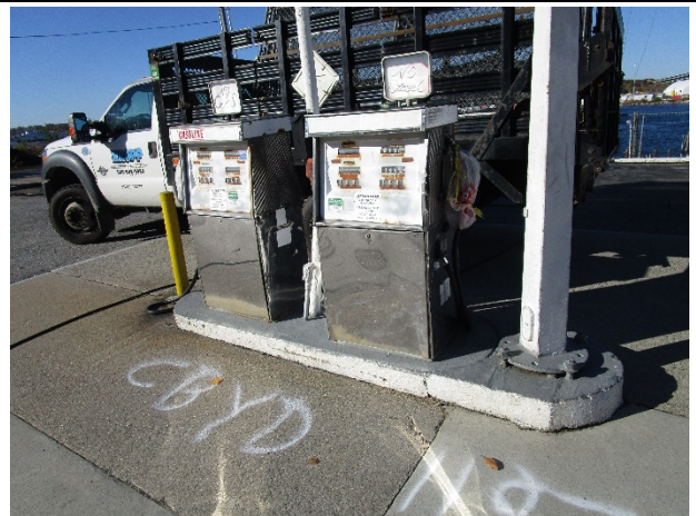
Photograph 2: Fuel Dispensers on Upper Portion of Site
