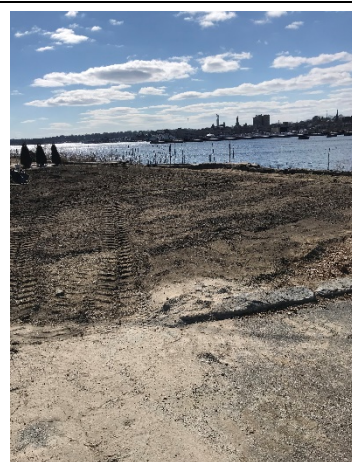
Photograph 24: UST Area after Backfilling
