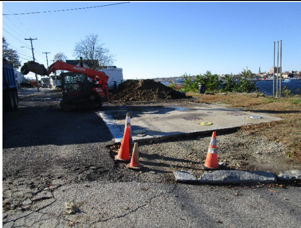
Photograph 1: UST Tank Pad
