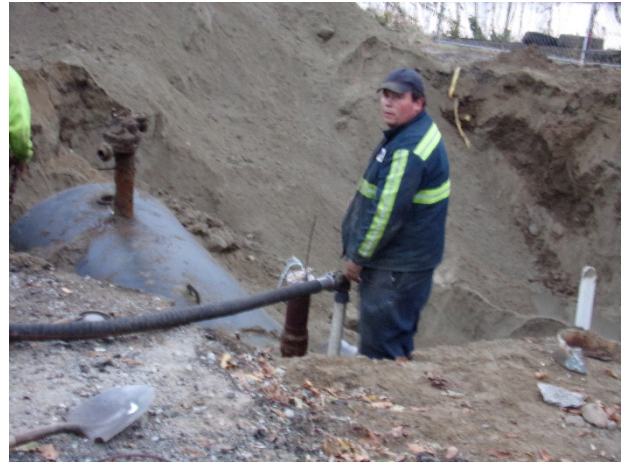
Photograph 16: Removing Residual Product from 2K Diesel Tank
