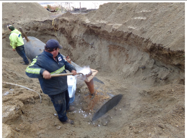
Photograph 10: Inerting Gasoline UST with Dry Ice
