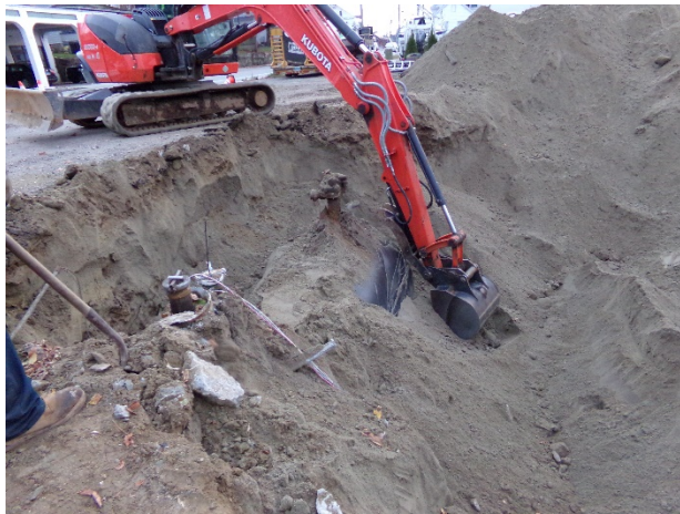
Photograph 15: Exposing 2K Diesel UST
