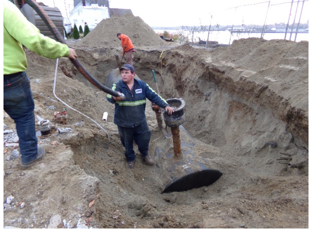
Photograph 8: Removing Residual Product from 4K Gasoline UST
