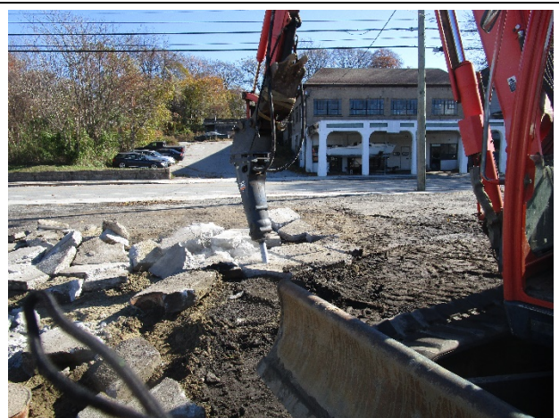
Photograph 4: Breaking up Concrete UST Pad
