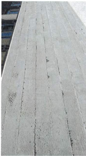
BOARD FORM FINISHED RETAINING WALL
