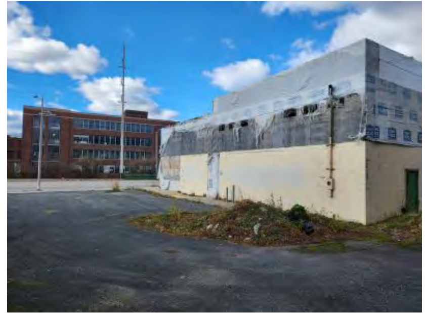
324 West Boylston St. – South Side (Looking NW)
