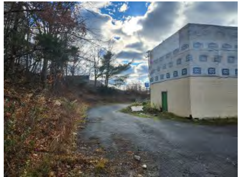
324 West Boylston St. – East Side (Looking South)
