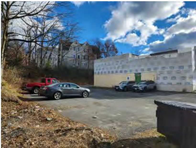
324 West Boylston St. – North Side (Looking SE)
