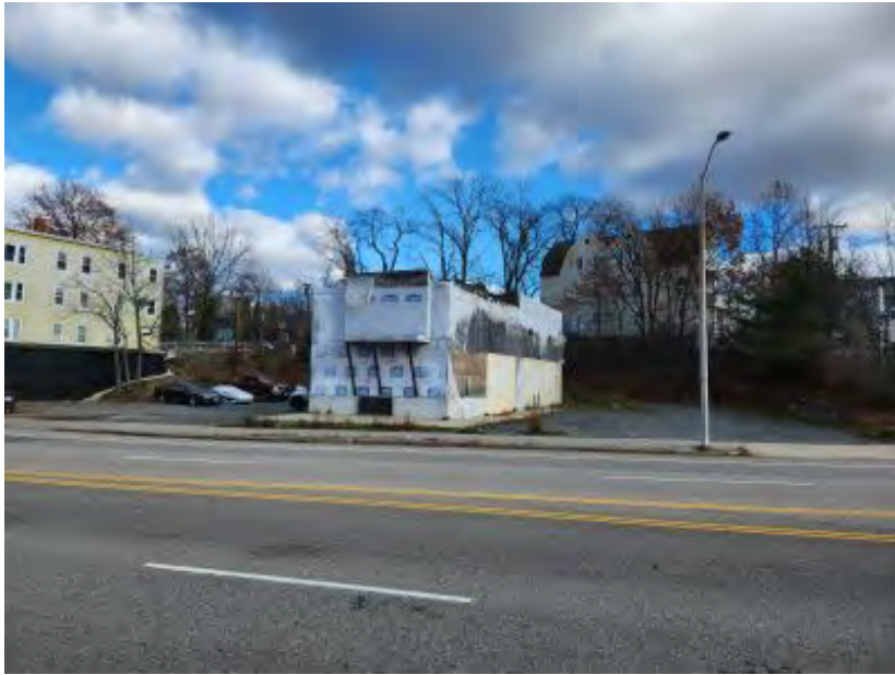
324 West Boylston St., Worcester, MA – Vacant (Looking ENE)
