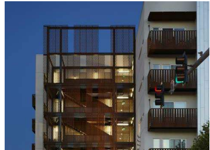
RETAIL / TEXTURED CONCRETE
