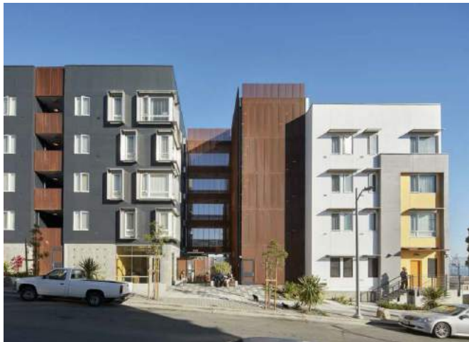
GROUND LEVEL / WOOD SIDING / TEXTURED CONCRETE
