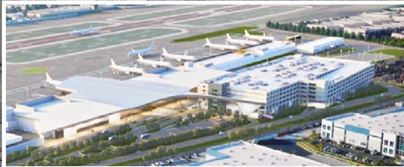
Burbank Airport Terminal Replacement
