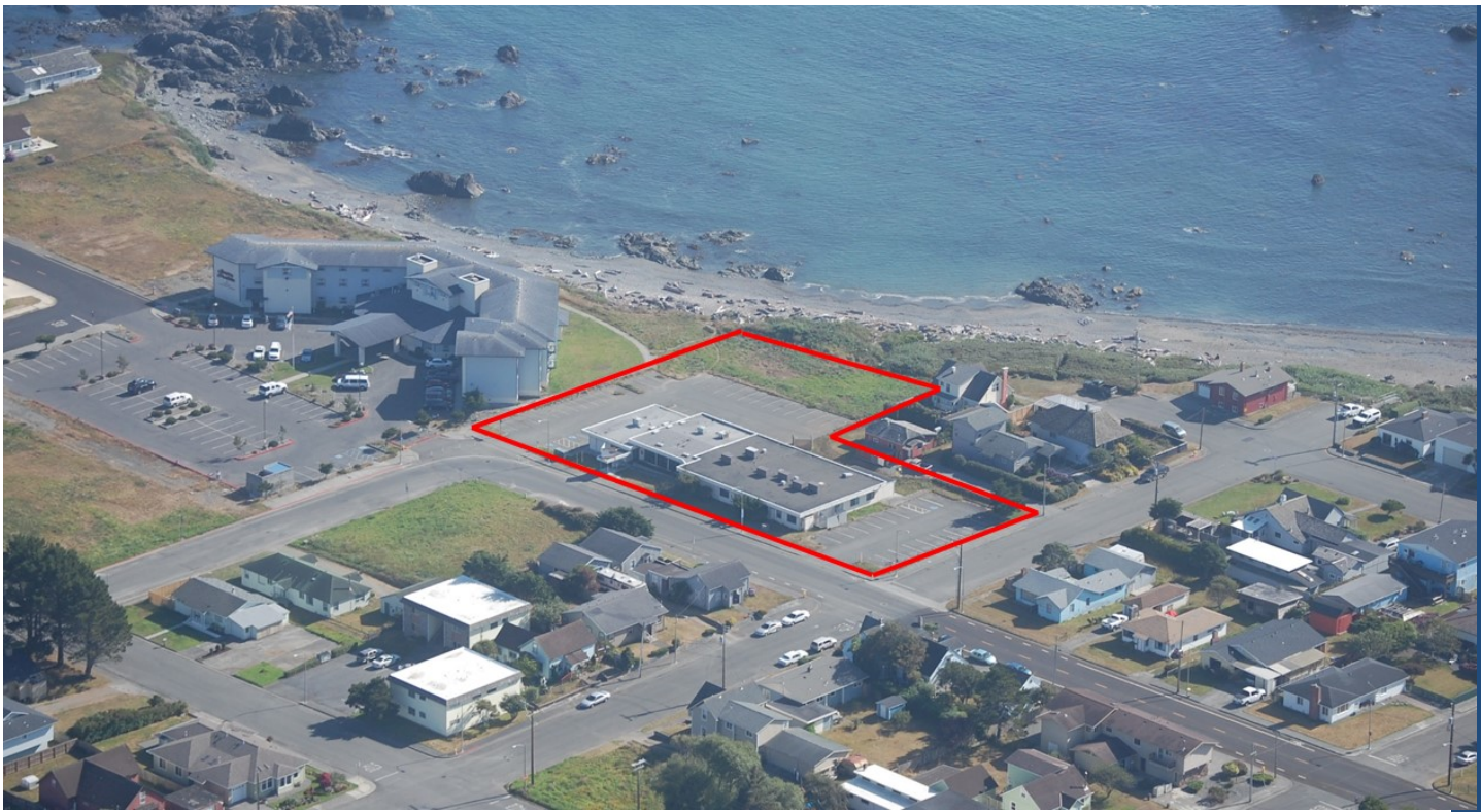
Beach Front , with direct access Unobstructed Views
